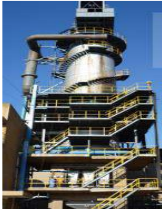
Figure 3.3: Four vertical ou four droit.
