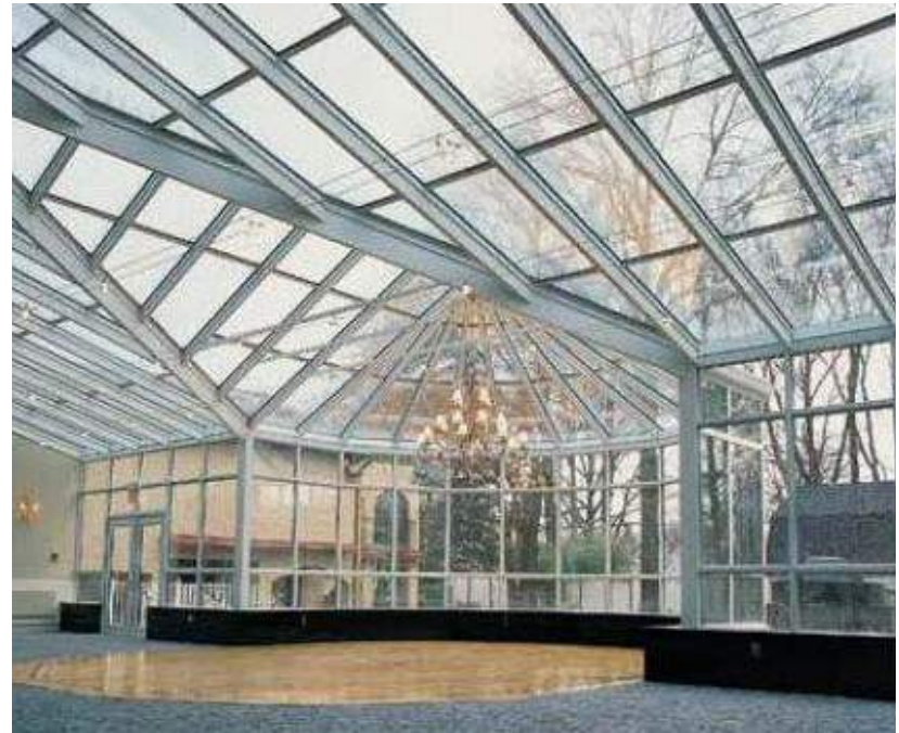
Photo courtesy of Four Seasons Solar Products LLC
