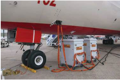
(a) Ground electrical power delivered to a Boeing 787. © Olivier Cleyner / Wikimedia Commons / CC-BY-SA-3.0.
