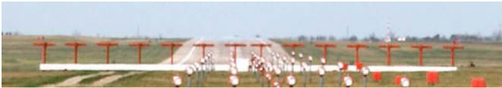
Figure 9.15: ILS: Localizer array and approach lighting. Wikimedia Commons / Public Domain.
