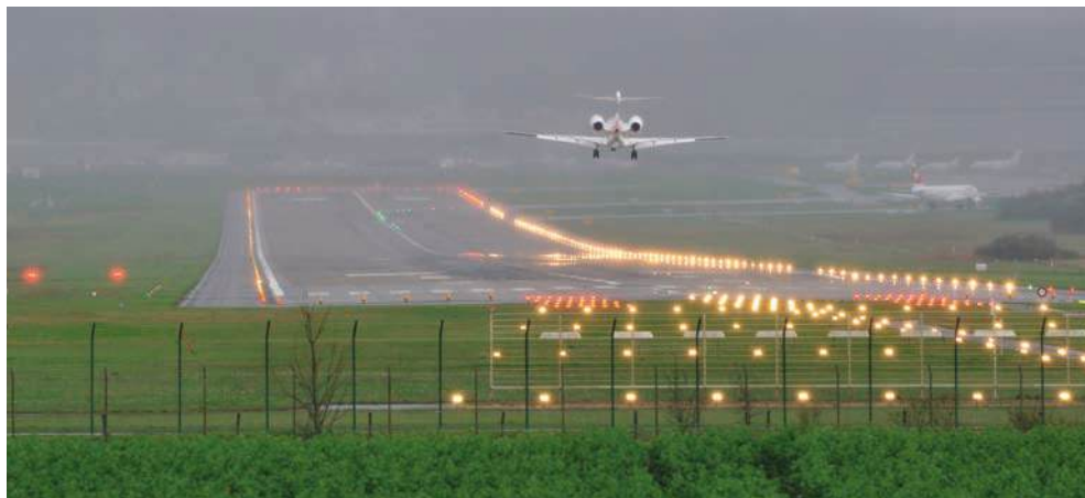
Figure 9.12: Runway lighting. © Hansueli Krapf / Wikimedia Commons / CC-BY-SA-3.0.
