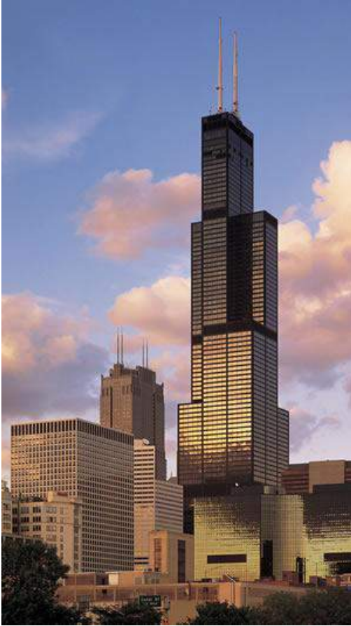
Fig. 4.95 – “Sears Tower” Building – Chicago, SUA
