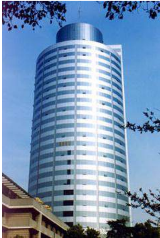
Fig. 4.108 – Building with curtain walls
