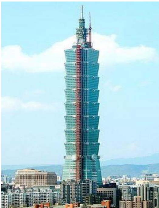
Fig. 4.97 – “Taipei 101” Tower – Taipei, Taiwan
