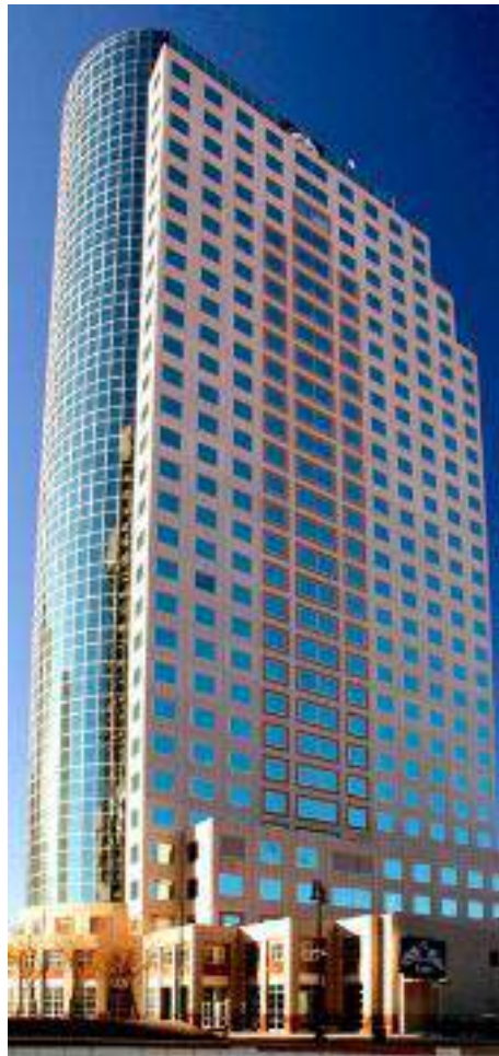
Fig.4.105 - The tallest building between Toronto and Calgary, Canwest. Constructed in 1990, the main tower structure is supported by a reinforced concrete core surrounded by perimeter steel framing and poured-in-place concrete decks.
