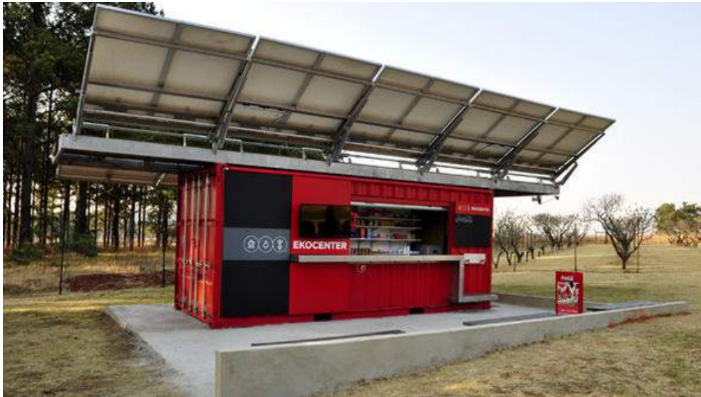
Figure 71: Clean Water Installation by Coca Cola
