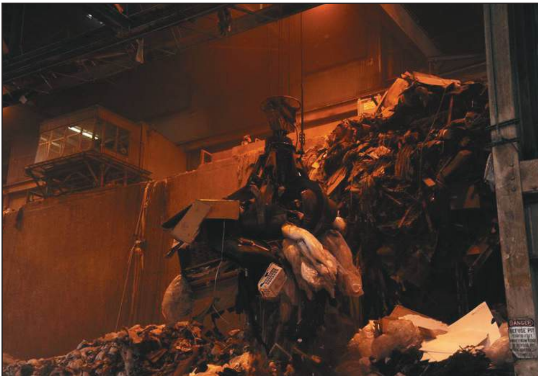
Figure 13.7 | The “Claw” moving plant waste and rubbish to incinerator
