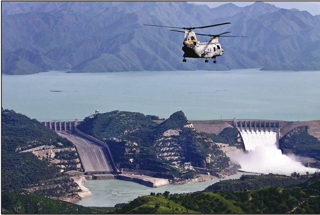
Figure 9.10 | World Bank Financed Tarbela Dam in Pakistan
