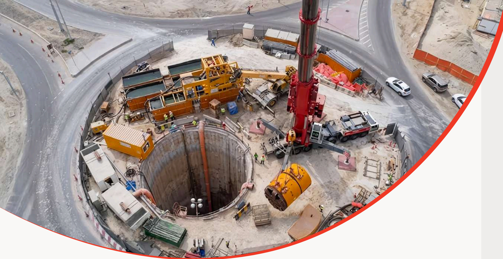
Secant Pile Work
