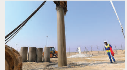
Secant Pile Work
