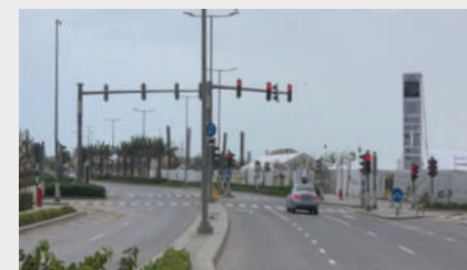
Street Lighting Network
