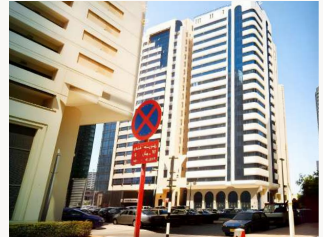
Al Rumaithy Building
