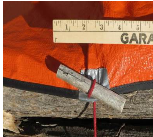
Figure 2: “Slip stick” for adjusting location of tarp ends during initial construction
