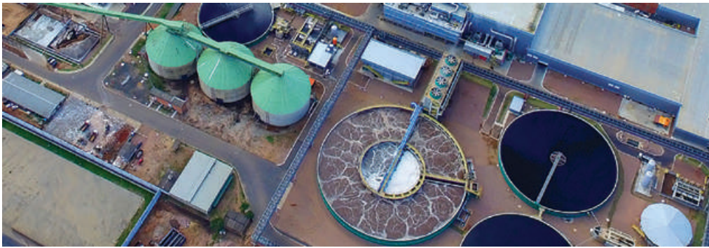
Figure 6.12 An activated sludge aeration basin (centre), clarifiers (right) and anaerobic digesters (left) used for treatment of high BOD wastewater from the pulp and paper industry. Image: Veolia Water Technologies/Wesley Santos/Agência PressDigital.
