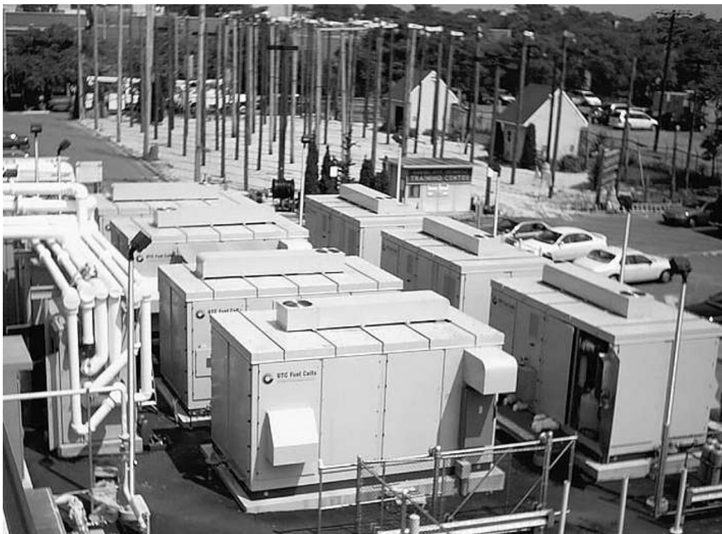
Fig. 7.17. In New York, U.S. the fuel cells from UTC Power generate 200 kilowatts each, providing a total of 1,4 megawatts of clean power (source: Image courtesy of UTC Power Corporation)
