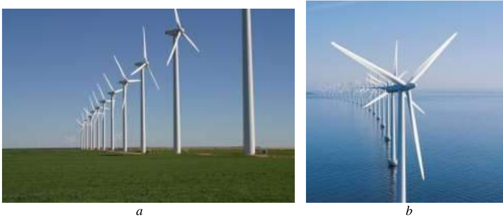
Fig. 7.12. Wind Power Plants: a) onshore (source: Creative Commons, Leaflet, 2004); b) offshore (source: IND Themes, GreenTechnology, 2013)
