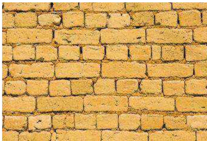
Fig. Brick work in mud
