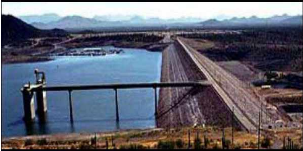
Fig. Non-overflow dam
