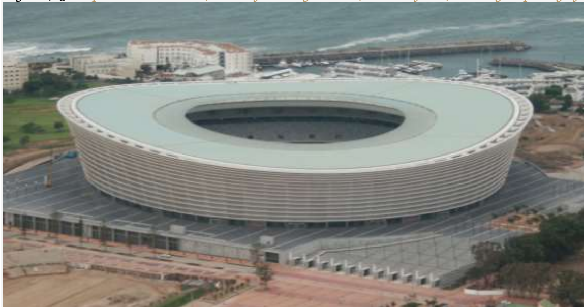
Figure 7.58 Cape Town Stadium, Taken from Signal Hill, South Africa; Seating Capacity of 64,100
