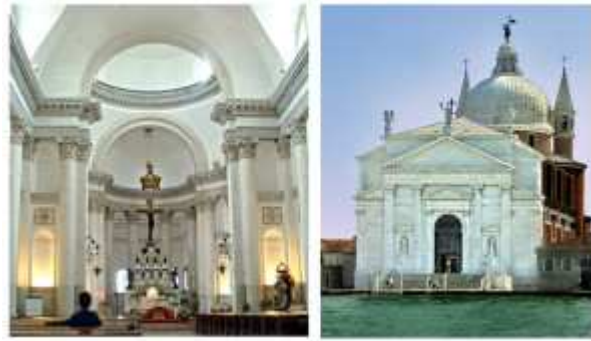
Fig. 8 The Italian Renaissance style makes use of antique columns, entablatures, cornices, niches, niches with statues, domes, round arches, temple-like fronts with pediments and tall attached columns or flat pilasters. The decoration in the interior is often restricted to a few contained shapes. A subtle limited palette of colors normally predominates. Pictured here is the interior and exterior of Il Redentore , in Venice; Andrea Palladio, begun ca. 1566
