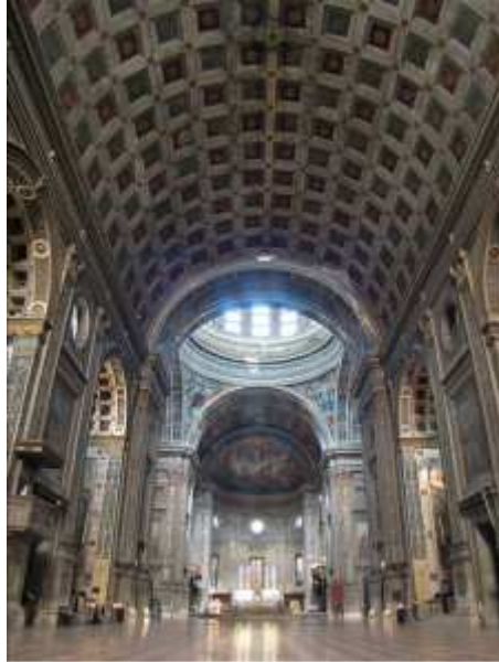
Fig. 14 The interior of Alberti's San Andrea with classical barrel vaults, dome and giant pilasters.
