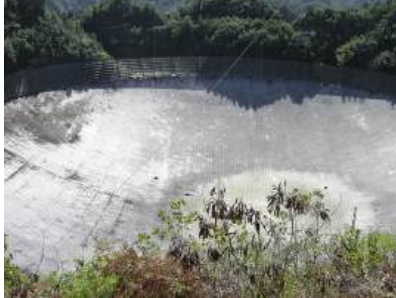
FIGURE 27.28 A 305-m-diameter natural bowl at Arecibo in Puerto Rico is lined with reflective material, making it into a radio telescope. It is the largest curved focusing dish in the world. Although D for Arecibo is much larger than for the Hubble Telescope, it detects much longer wavelength radiation and its diffraction limit is significantly poorer than Hubble's. Arecibo is still very useful, because important information is carried by radio waves that is not carried by visible light. (credit: Tatyana Temirbulatova, Flickr)
