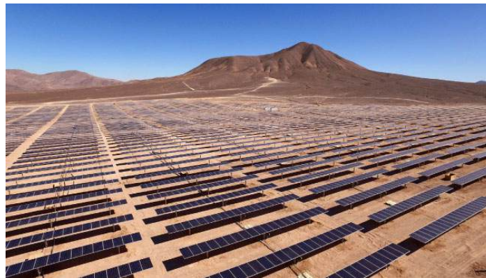
FIGURE 7.28 Solar cell arrays at a power plant in California (credit: Bureau of Land Management, Flickr)
