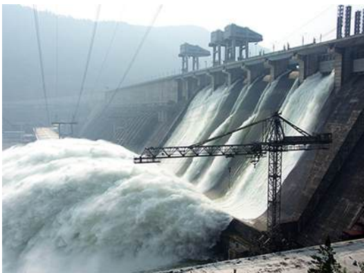
FIGURE 7.35 Hydroelectric facility (credit: Denis Belevich, Wikimedia Commons)
