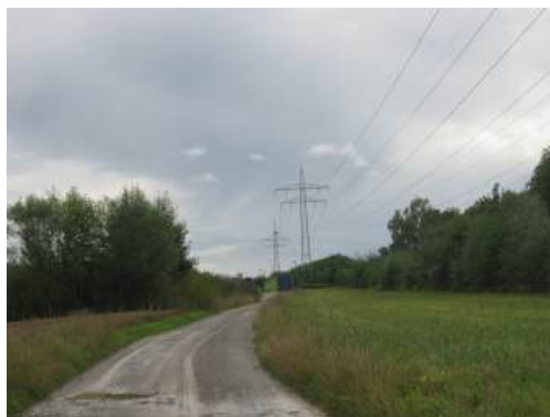
FIGURE 24.9 This high-voltage traction power line running to Eutingen Railway Substation in Germany radiates electromagnetic waves with very long wavelengths. (credit: Zonk43, Wikimedia Commons)
