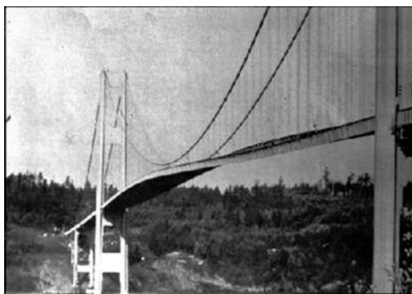
FIGURE 16.26 In 1940, the Tacoma Narrows Bridge in Washington state collapsed. Heavy cross winds drove the bridge into oscillations at its resonant frequency. Damping decreased when support cables broke loose and started to slip over the towers, allowing increasingly greater amplitudes until the structure failed (credit: PRI's Studio 360 , via Flickr)
