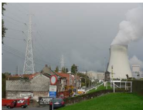
FIGURE 32.20 The people living near this nuclear power plant have no measurable exposure to radiation that is traceable to the plant. About 16% of the world's electrical power is generated by controlled nuclear fission in such plants. The cooling towers are the most prominent features but are not unique to nuclear power. The reactor is in the small domed building to the left of the towers. (credit: Kalmthouts)
