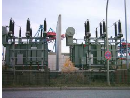
FIGURE 20.17 Power is distributed over large distances at high voltage to reduce power loss in the transmission lines. The voltages generated at the power plant are stepped up by passive devices called transformers (see Transformers ) to 330,000 volts (or more in some places worldwide). At the point of use, the transformers reduce the voltage transmitted for safe residential and commercial use. (Credit: GeorgHH, Wikimedia Commons)
