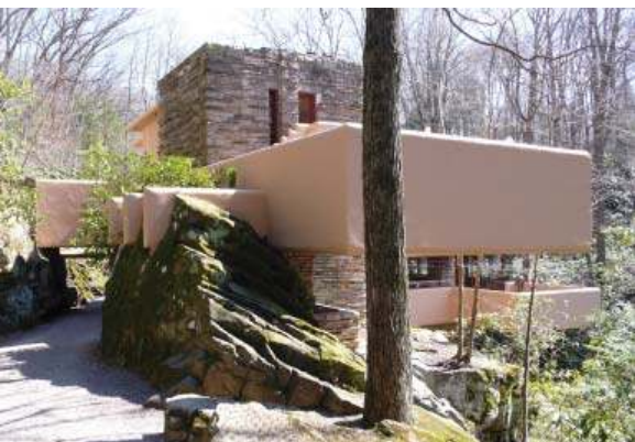
Fig. 5.5.6 The North side of the house is securely embedded into the existing hill-side and boulders, creating a strong earthly tie to the site.
