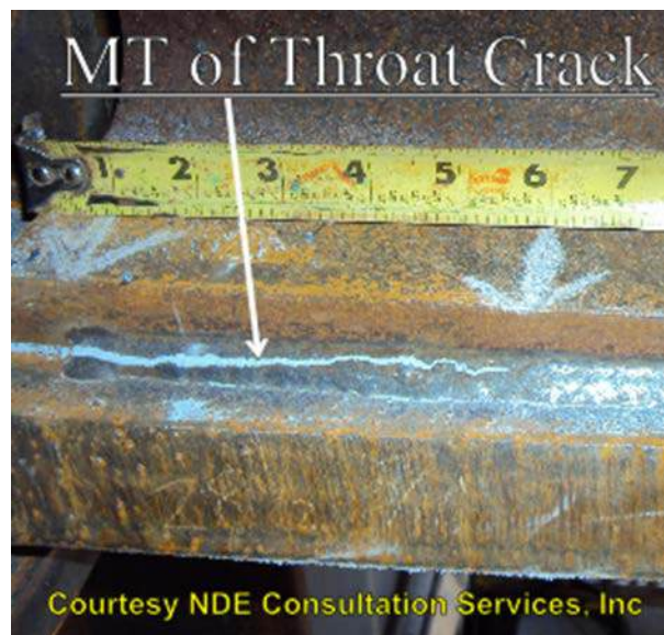
Figure 20: MT of throat crack
