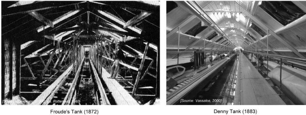
Figure 1.3: The World's First Towing Tanks
