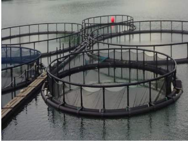
Plate 2.1 Circular cages made of HDPE pipes
