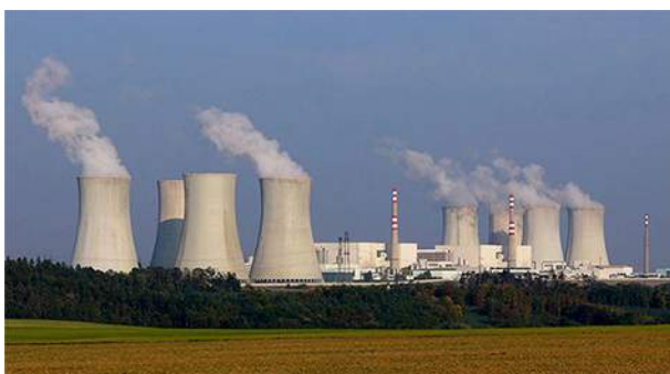
Figure 4.5 The heat exhausted from a nuclear power plant goes to the cooling towers, where it is released into the atmosphere.
