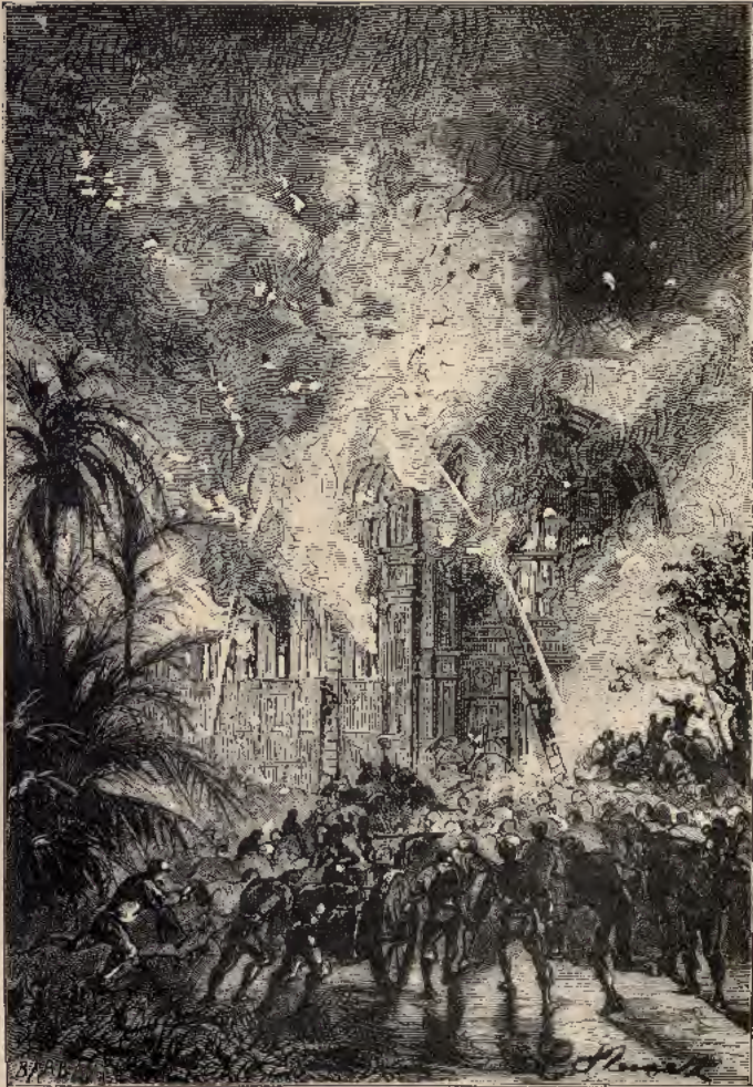
A destructive fire.
