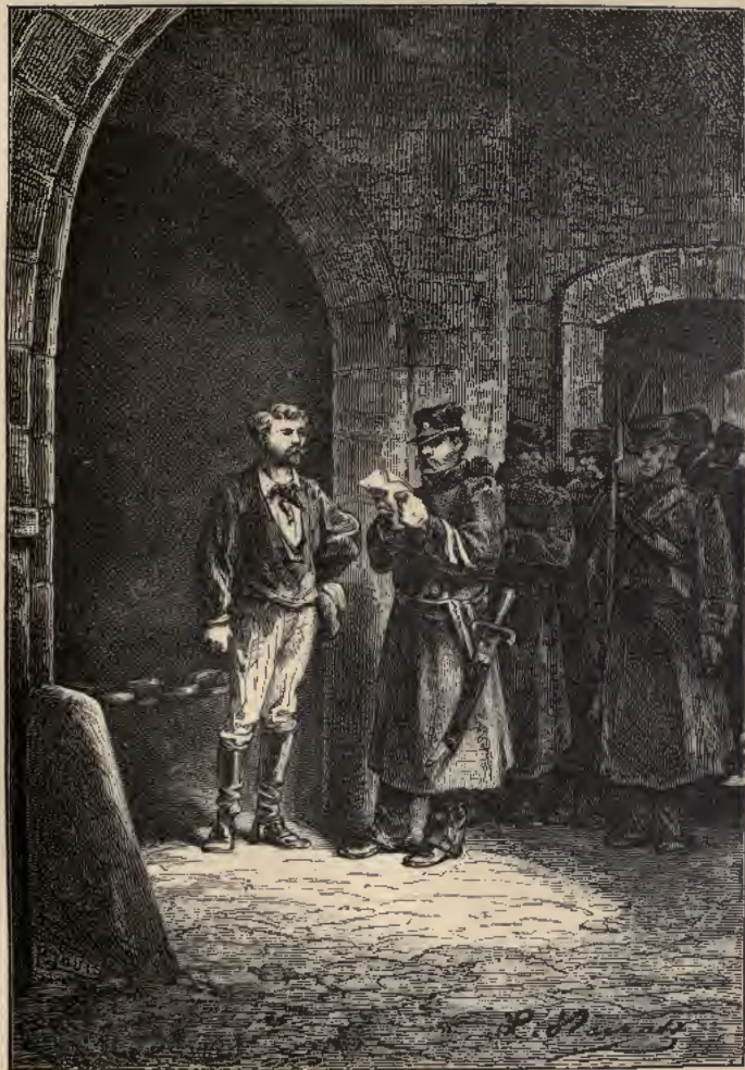
The new workman.
