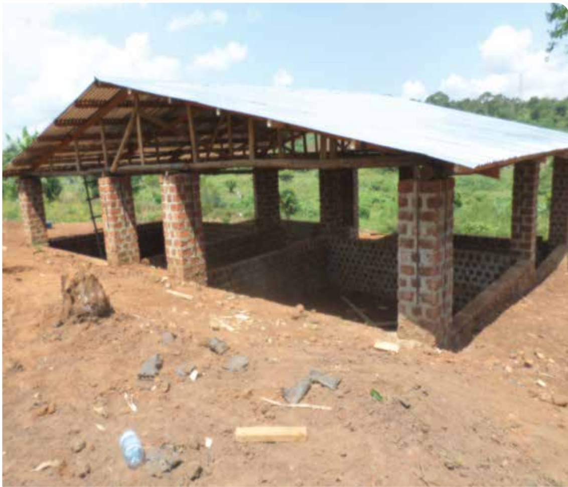
Figure 20 four unit FBT piggery housing structure before plastering of walls was done.
