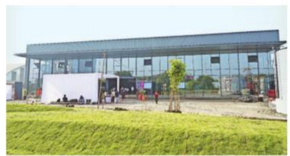
Construction work underway on Deakin campus. Express
