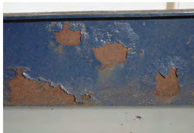
Figure 2 Detail of One for Bristol , indicating paint loss and corrosion in 2010. © The Artist's estate.
