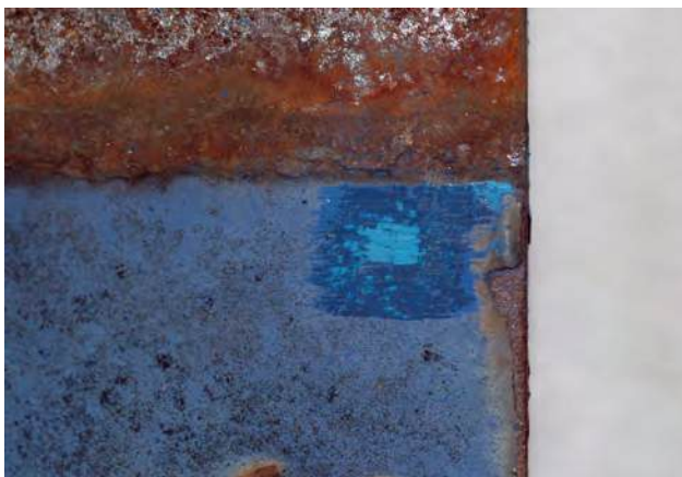
Figure 3 Detail of One for Bristol . A scratch test revealed the original paint finish underneath.
