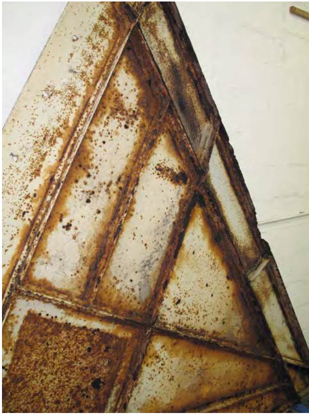
Figure 6 Reverse face of water-damaged painted steel. Pristine paint is not just an aesthetic consideration. Failing paint layers can quickly lead to water penetration. On steel sculptures, this can result in rusting and structural weakness. Photo: Tom Learner.
