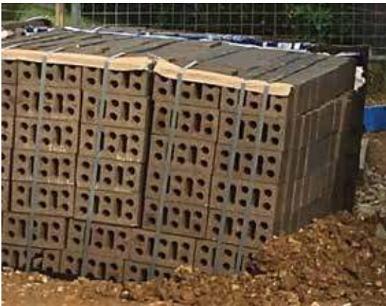
Figure 9 – Example of poor brick storage
