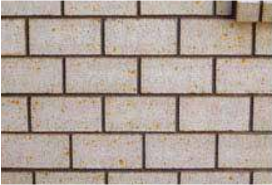
Figure 5 – Iron Staining on Brick Faces
