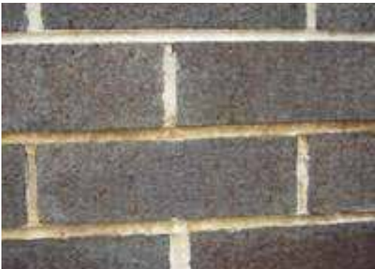
Figure 6 – Iron Staining in Mortar Joints
