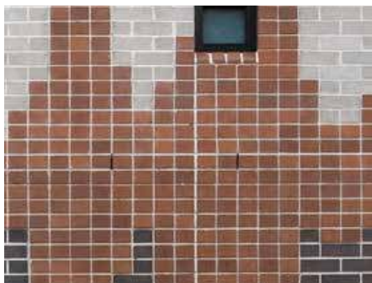
Figure 5 – Control Joint
