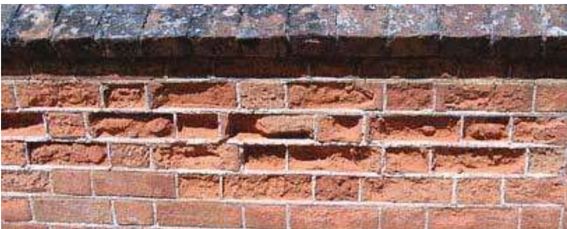
Figure 3 – Effect of salt attack on brickwork
