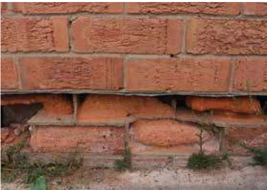
Figure 1 – Salt attack damage to masonry unit
