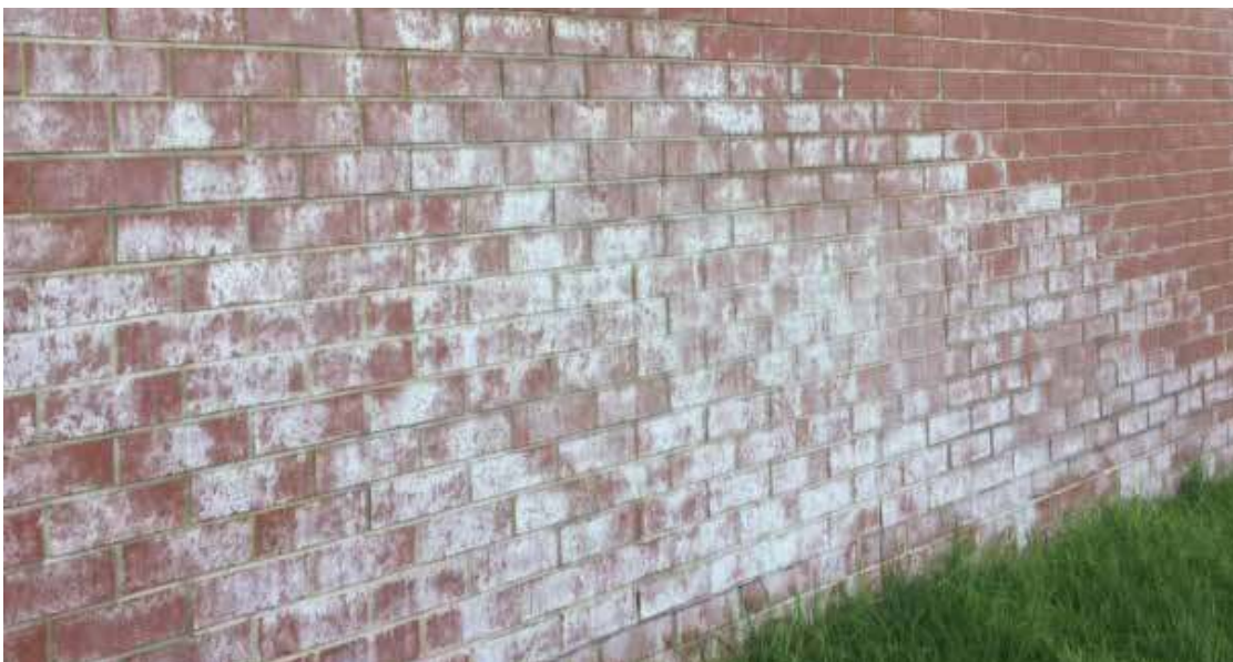
Figure 3 – Efflorescence on brickwork
