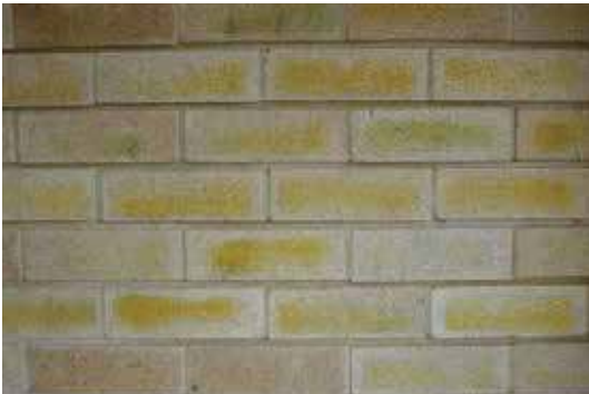
Figure 7 – Vanadium staining on brick face
