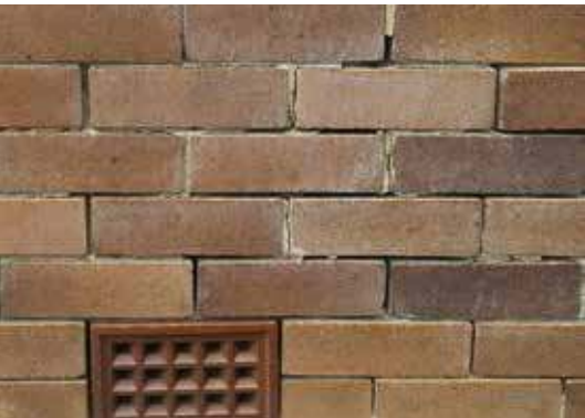
Figure 2 – Salt attack damage to mortar
