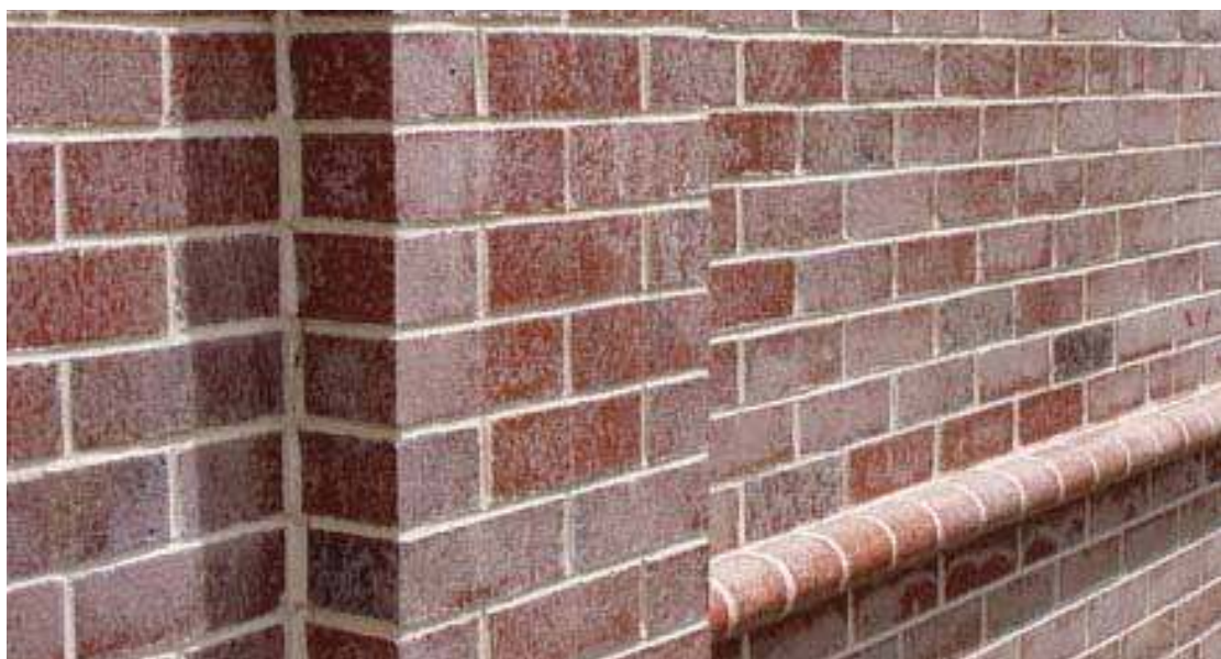
Figure 4 – Brickwork effected by efflorescence
