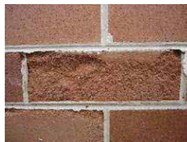
Figure 1 – Dry press brick damage due to high pressure cleaning
