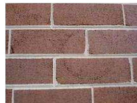
Figure 2 – Damage resulting from the use of a turbo head
