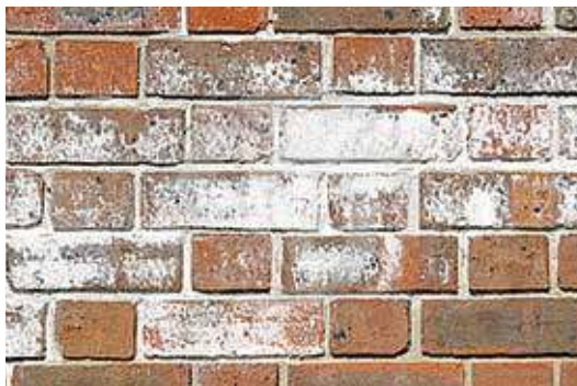
Figure 4 – Insoluble white deposits on brickwork
