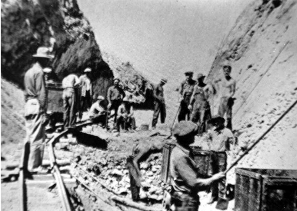
Figure 2. WPA laborers remove overburden (NPS photo).
