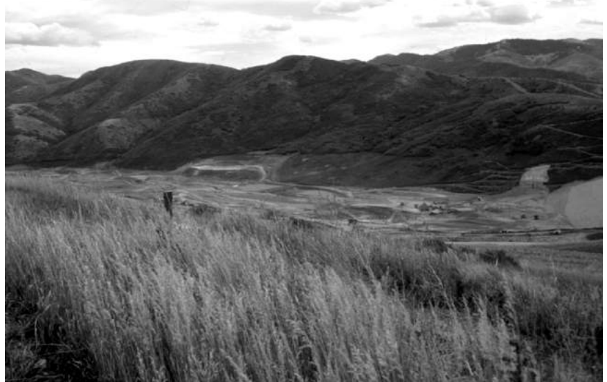
Figure 1. Overview of the Little Dell Reservoir excavation.
