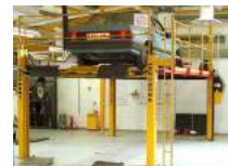
Four post lift in use Two post lift
