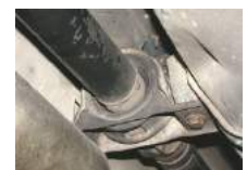
This bearing prevents propshaft whip
