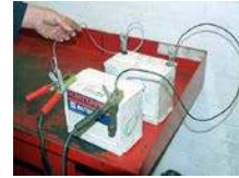
Connecting batteries in parallel (12 V)
