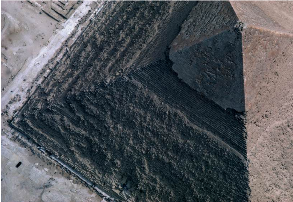
Fig. 6. Aerial view of the casing stones and upper levels of the Pyramid of Khafre. With permission © Kazuyoshi Nomach. The upper layers of this pyramid indicate that a more sophisticated construction method may have been used as the height increased and the summit was approached. A fairly clear horizontal line separates two possible zones of construction.
