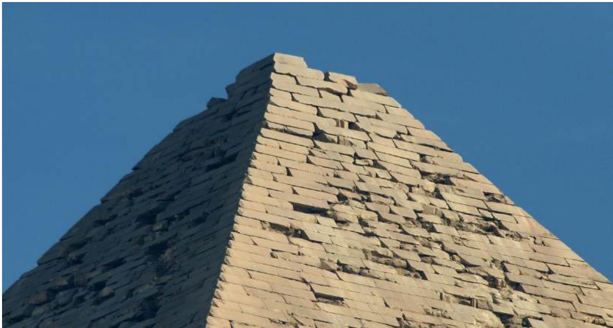
Fig. 5. Casing stones still in situ near the summit of the Pyramid of Khafre at Giza, showing a high degree of regularity which may have contributed to their structural integrity and survival. With permission © Franck Monnier.
