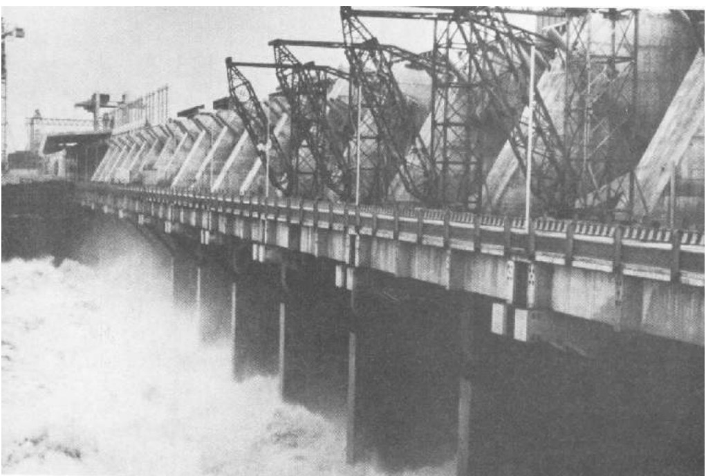
Salto Grande hydroelectric dam Photos courtesy Inter-American Development Bank
