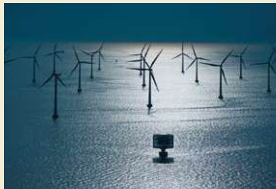
7.12 e > Offshore wind turbines produce electricity in many places around the world. One of the largest offshore wind farms, consisting of 48 turbines, is located in the Baltic Sea between Denmark and Sweden. A transformer station has been constructed here to feed power into the Swedish grid.
