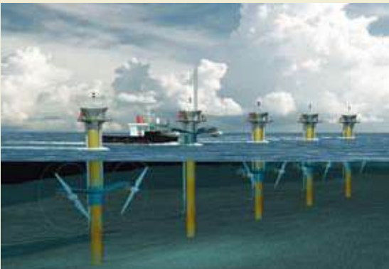
7.12 b > Tidal energy can be converted to electricity by underwater rotors, as at the SeaGen plant off the coast of Northern Ireland in Strangford Lough. One facility has already been constructed which feeds electricity into the grid onshore. Others will follow.
