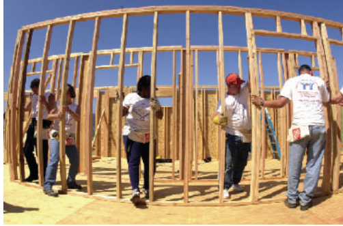
FIGURE 1.10 After the Southern California wildfires in 2003, sailors from the USS Ronald Reagan helped volunteers rebuild houses in San Pasqual as part of Habitat for Humanity. Habitat for Humanity builds homes for low-income people. (credit: Johansen Laurel, U. S. Navy)
