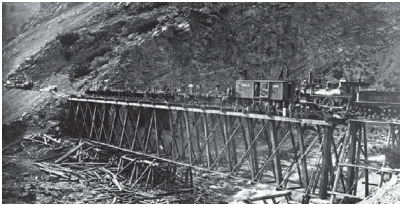
FIGURE 16.6 In an example of distributive policy, the Union Pacific Railroad was given land and resources to help build a national railroad system. Here, its workers construct the Devil's Gate Bridge in Utah in 1869.
