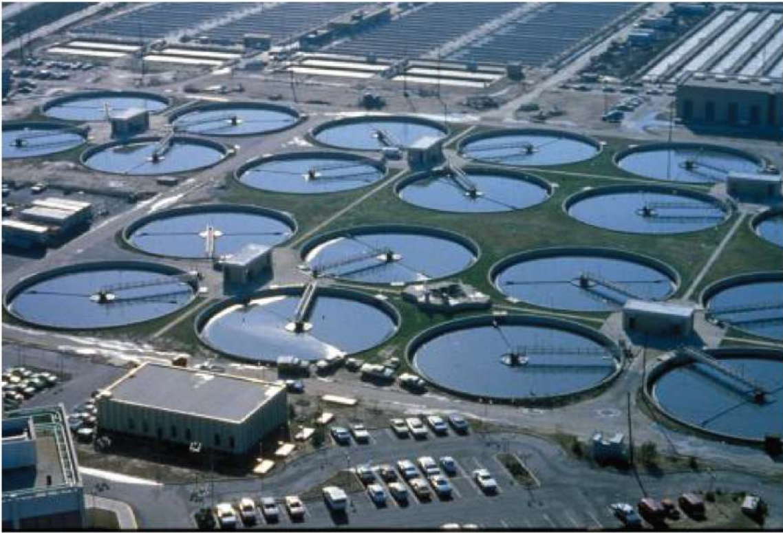
Figure 25.0 Sewage Treatment Plant. (credit: "eutrophication&hypoxia"/flickr.com)
