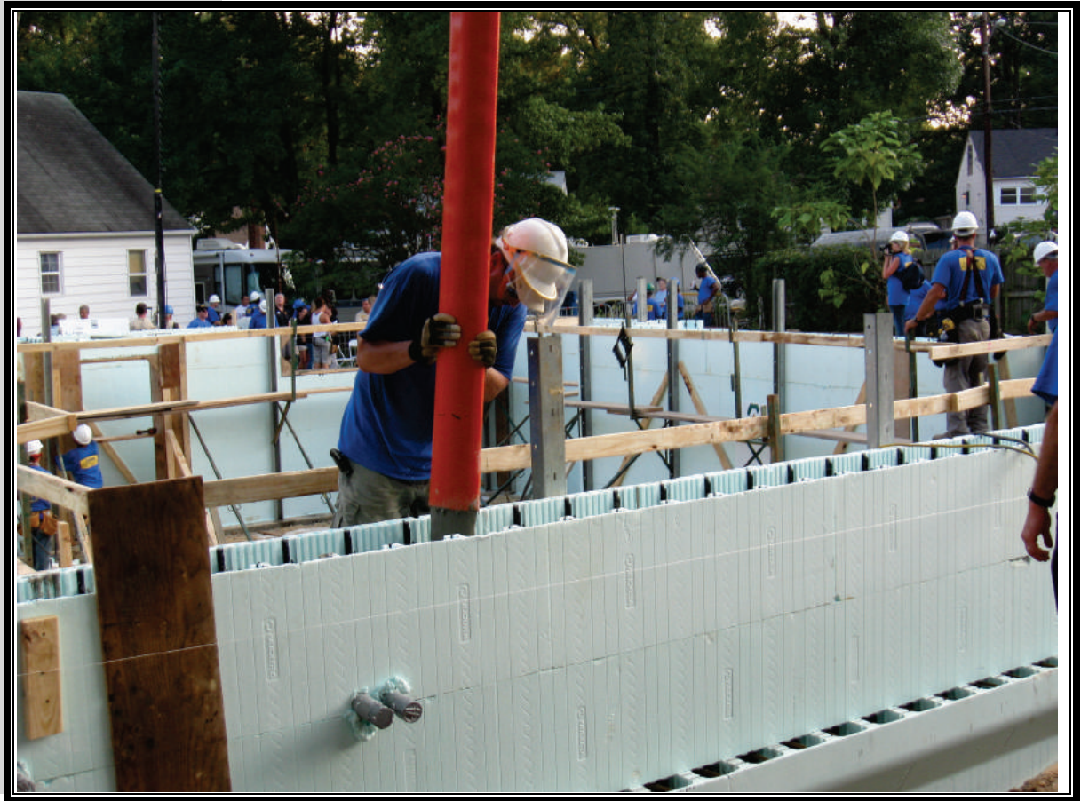
House Construction Using Insulating Concrete Forms
