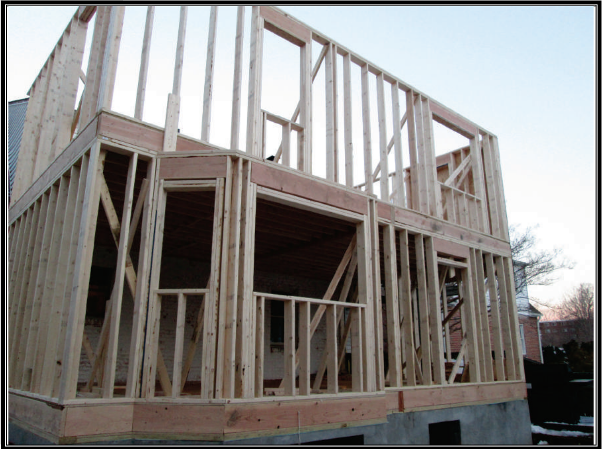
Modern Platform-Framed House Under Construction
