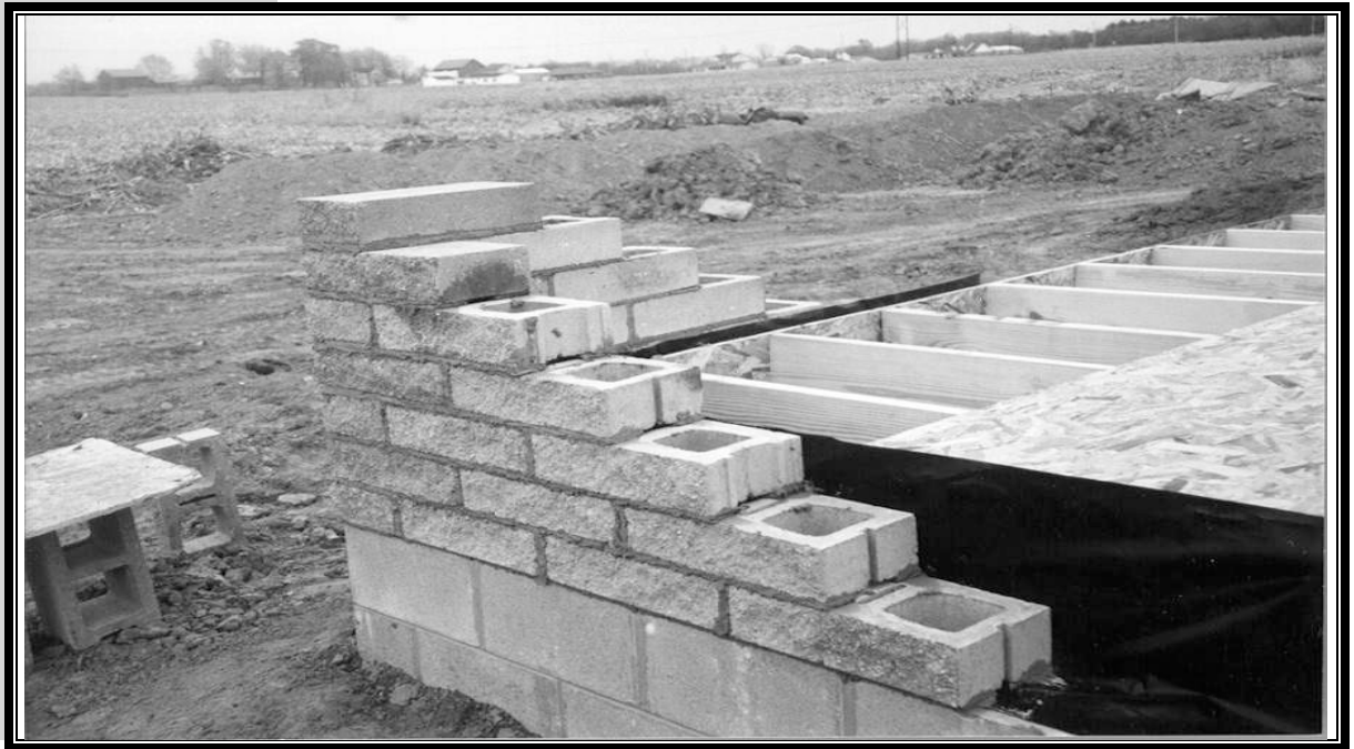
FIGURE 1.6 House Construction Using Concrete Masonry
