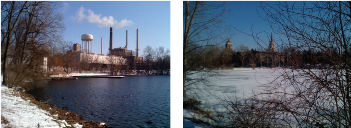
Figure 4.25: St. Joseph's Lake (left) and St. Mary's Lake (right) on the University of Notre Dame campus, 14 February 2010, demonstrating the effect of exchanging heat with the condenser of the Notre Dame power plant near St. Joseph's Lake.
