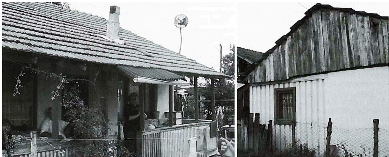
Figure 1.23 - (Left) Front view of the house; (Right) Side view of the housing showing the shipping container, Duzce, Turkey (Source: Book “Rebuilding after disasters” (Lizarralde et al., 2010))
