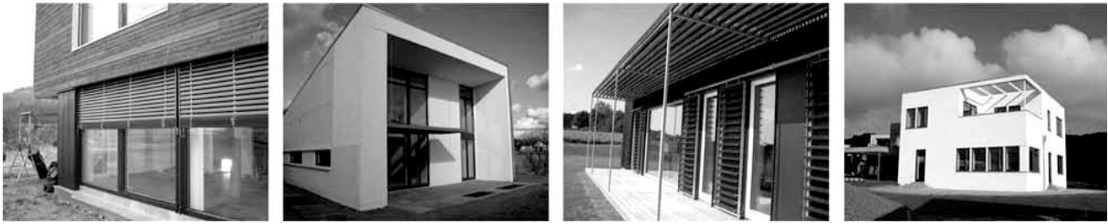
Figure 4.3- External shading. (Left to right: a., b., c. d., respectively) (Source: (Velux Group, 2010))
