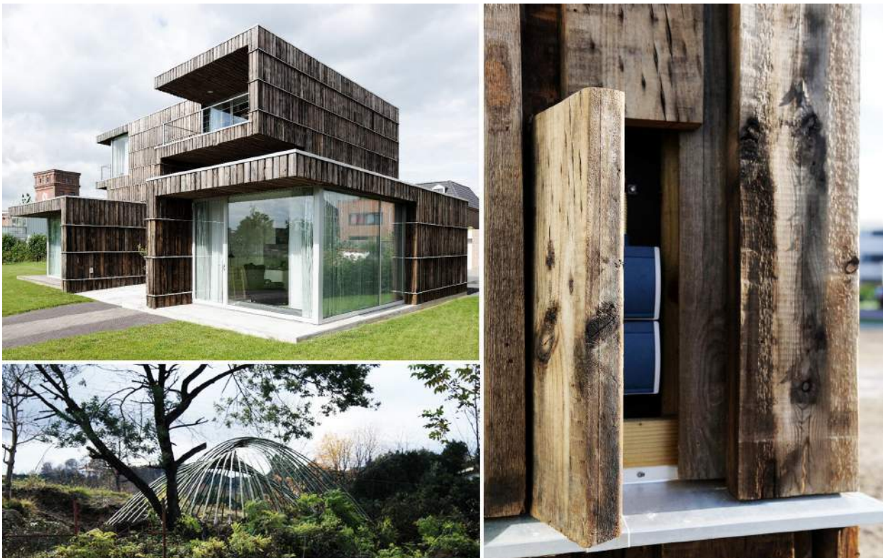
Figure 1.21 – (Left above and Right) Villa Welpeloo a house mainly built out of demolition materials and manufacturing residues. It is a smart example of how the topic of recycling can be developed into a unique and elegant architectural style. To decrease the carbon footprint even more, all the materials were sourced within a nine mile radius of where the home stands. Through a process the architects call recyclicity (rather than the more commonly used term of salvaging), 60% of the exterior and nearly 90% of the interior are composed of reused and repurposed materials. (Left below) Sustainable Bamboo Dome : The base of the self-standing shelter was made from gas pipes from a local shop, ensuring the structure can be move to another location if required (Source: Villa Welpeloo: http://www.archello.com/en/project/villa-welpeloo ; Dome: http://inhabitat.com/iranian-architect-builds-sustainable-bamboo-dome-from-bamboo-and-dry-rice-plants/pouya-khazaeli-parsa-bamboo-and-rice-dome-iran-2/?extend=1 )
