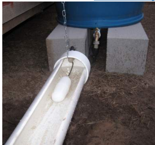
Figure 6-13: Automatic Watering System
