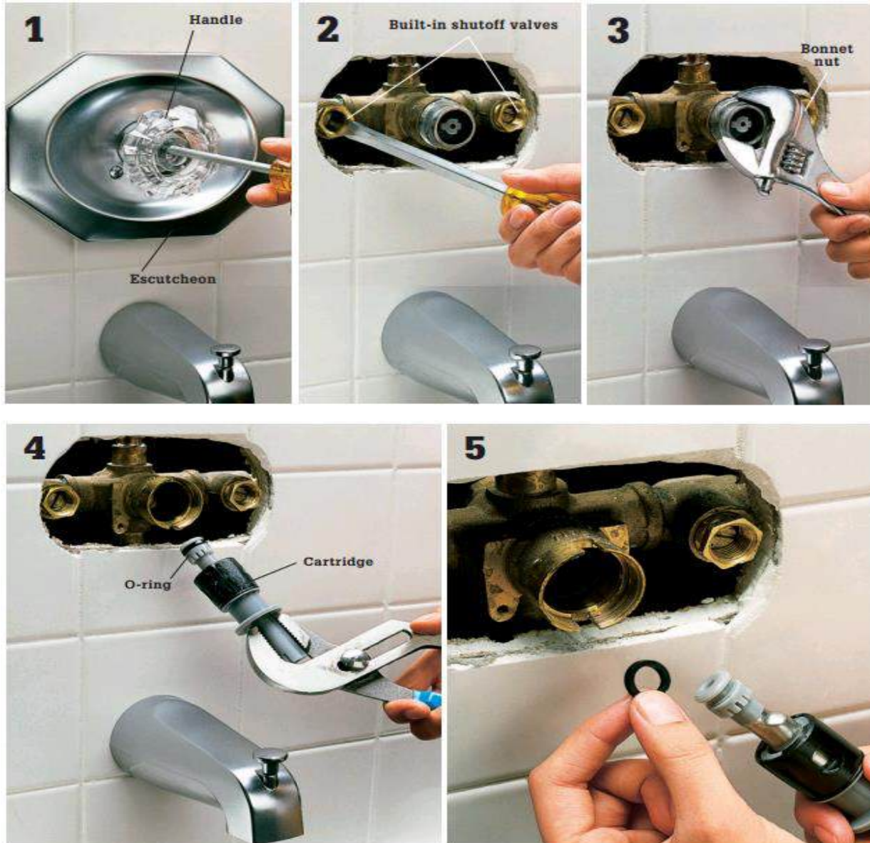
Figure 3.73 Repair a Single-handle Cartridge Tub and Shower Faucet
