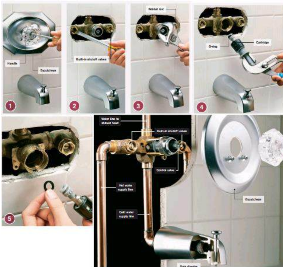
Figure 3.72 Fixing Single-Handle Tub & Shower Faucets
