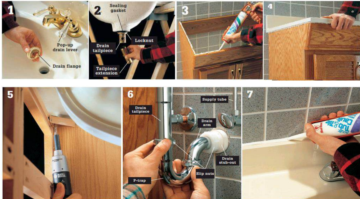
Figure 3.85 Installing an Integral Vanity Top
