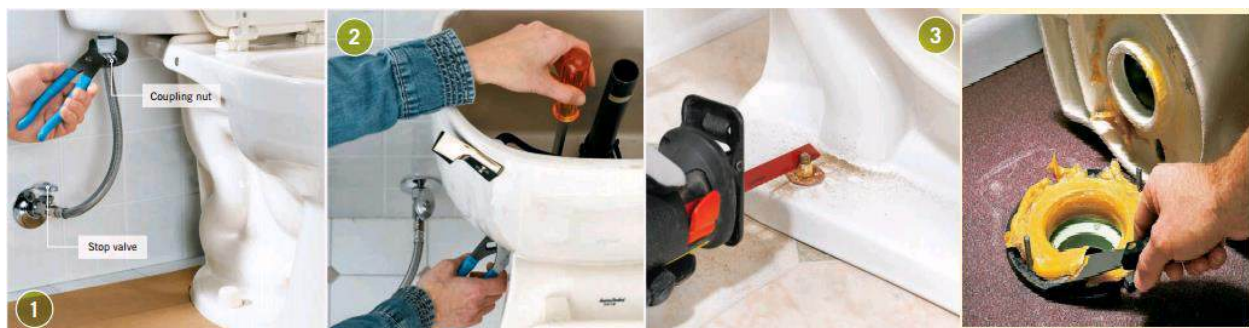
Figure 3.55 Steps to Repair water closet
