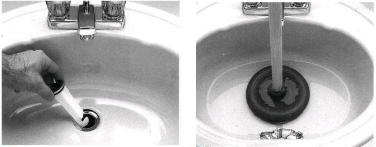
Figure 3.96 Clear Sink Drains with a Plunger
