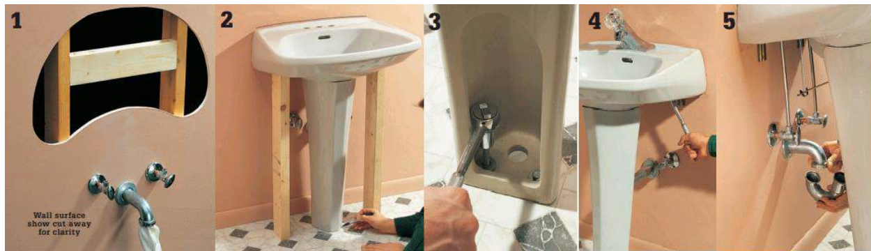
Figure 3.27 Install a Pedestal Sink
