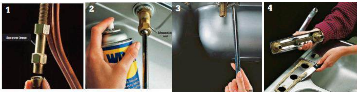
Figure 3.98 Maintaining and Repairing of Sink faucet
