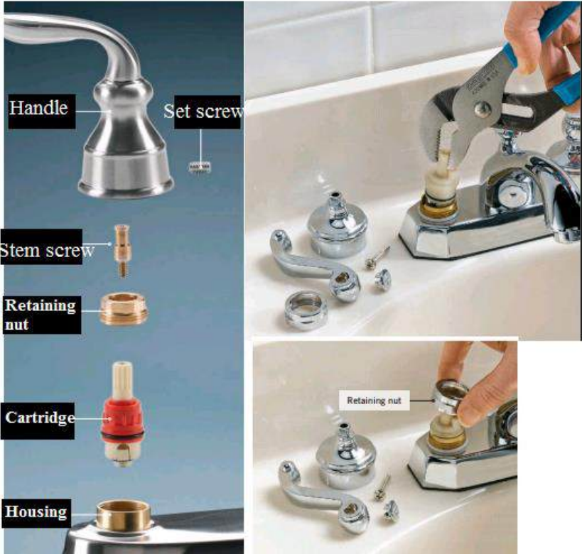
Figure 3.88 Washerless Two-Handle Faucet
