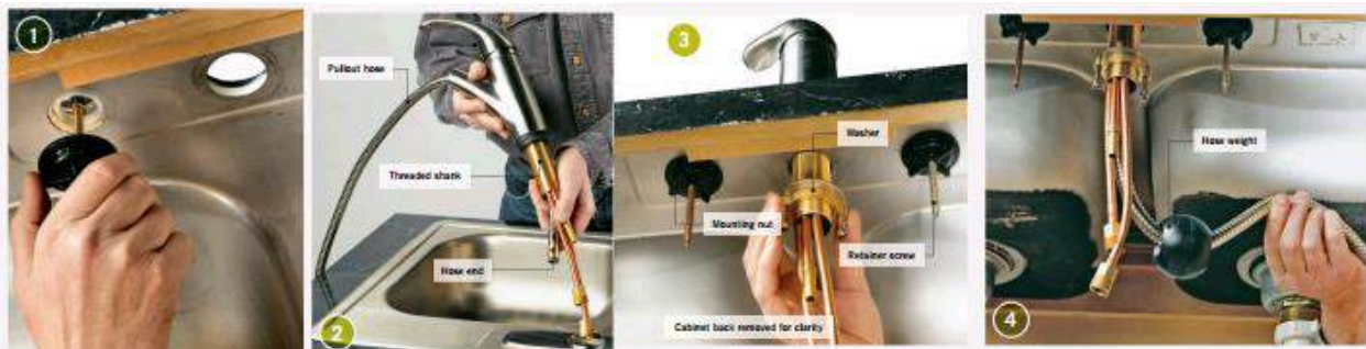
Figure 3.81 Steps of Installation of sink
