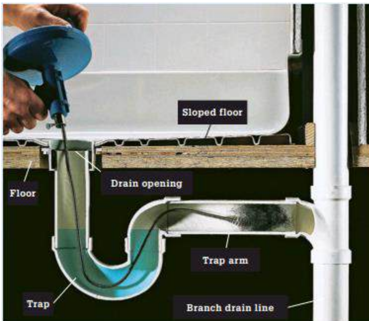
Figure 3.66 Clearing of Shower pan installation
