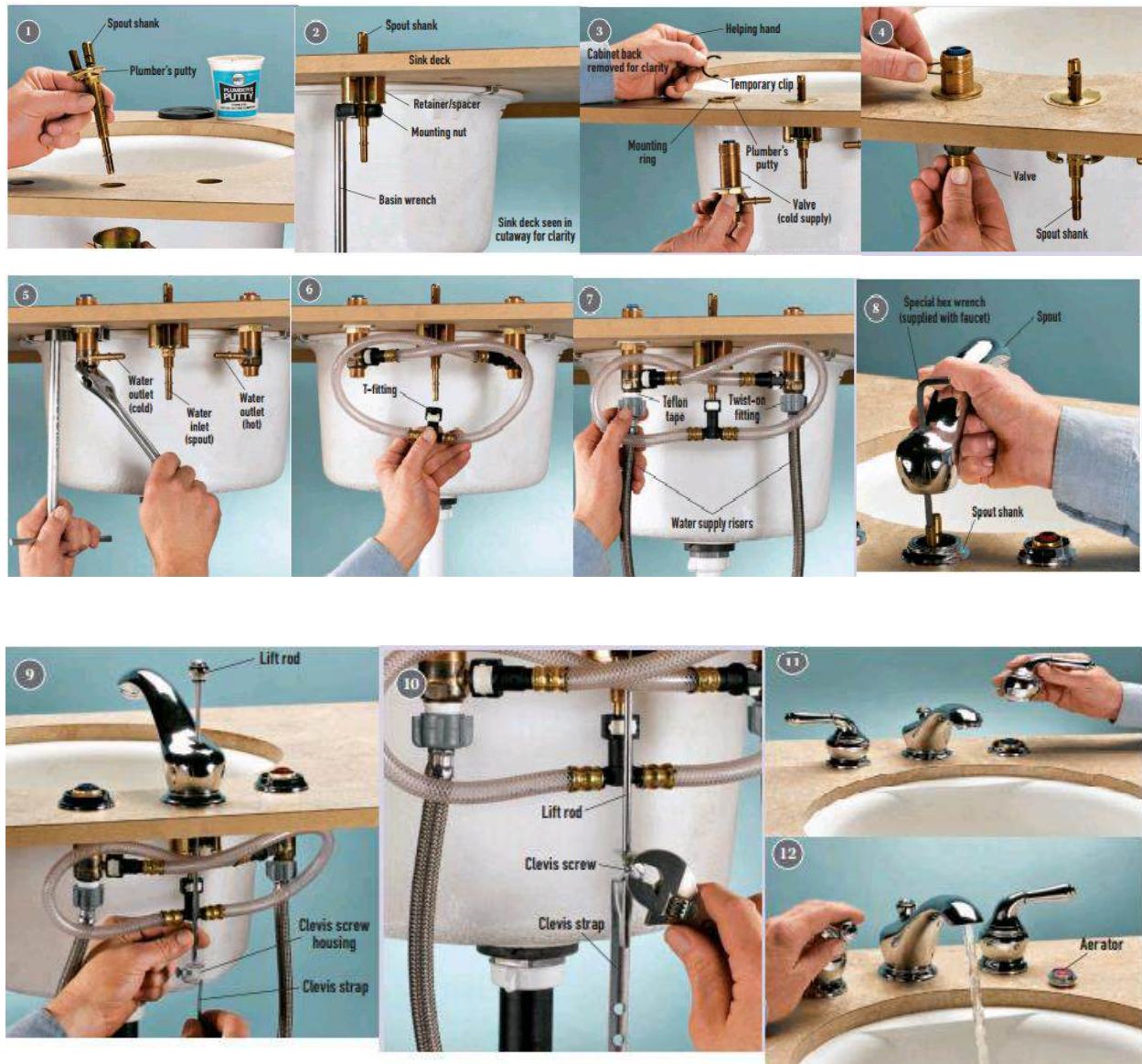
Figure 3.31 Installing a widespread faucet
