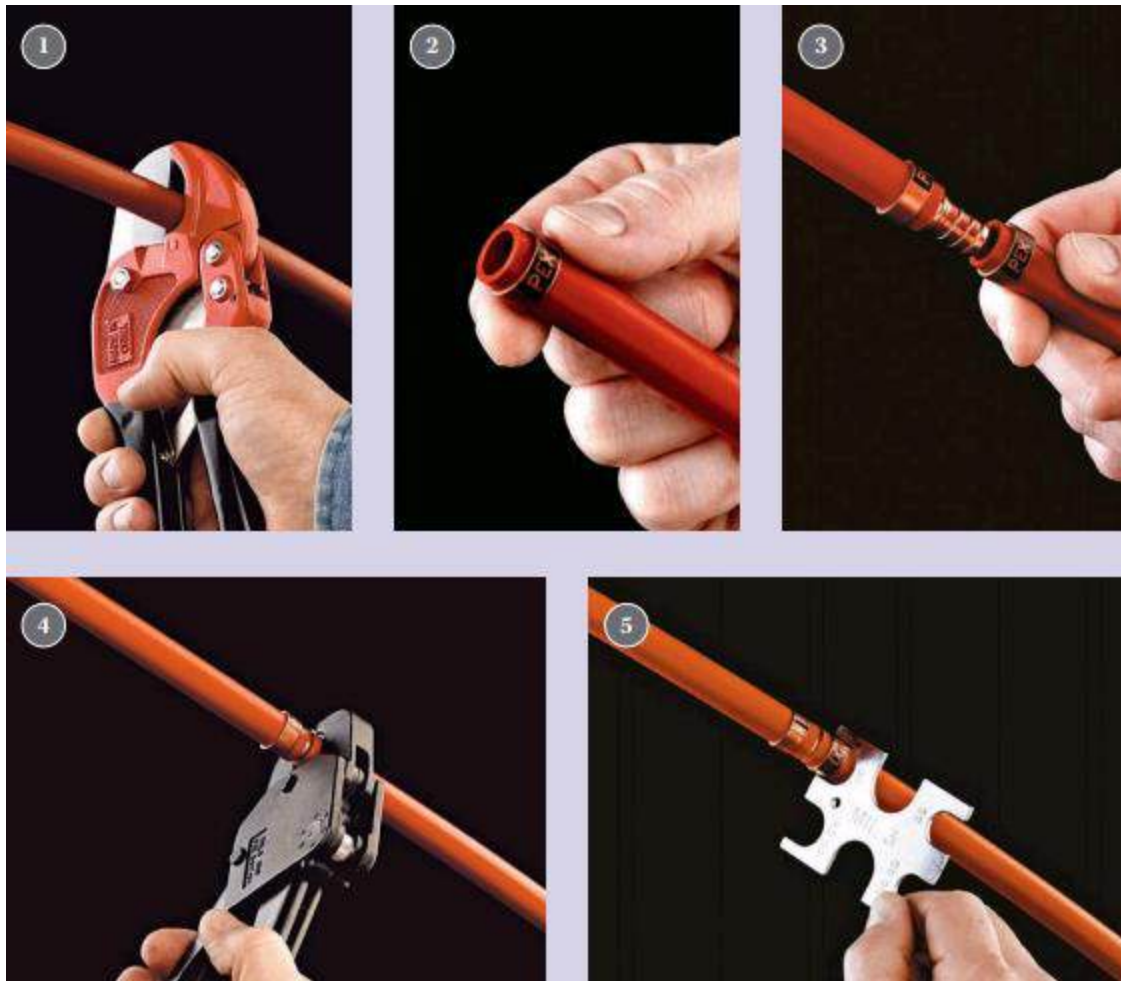
Figure 2.42 Steps of installing PEX
