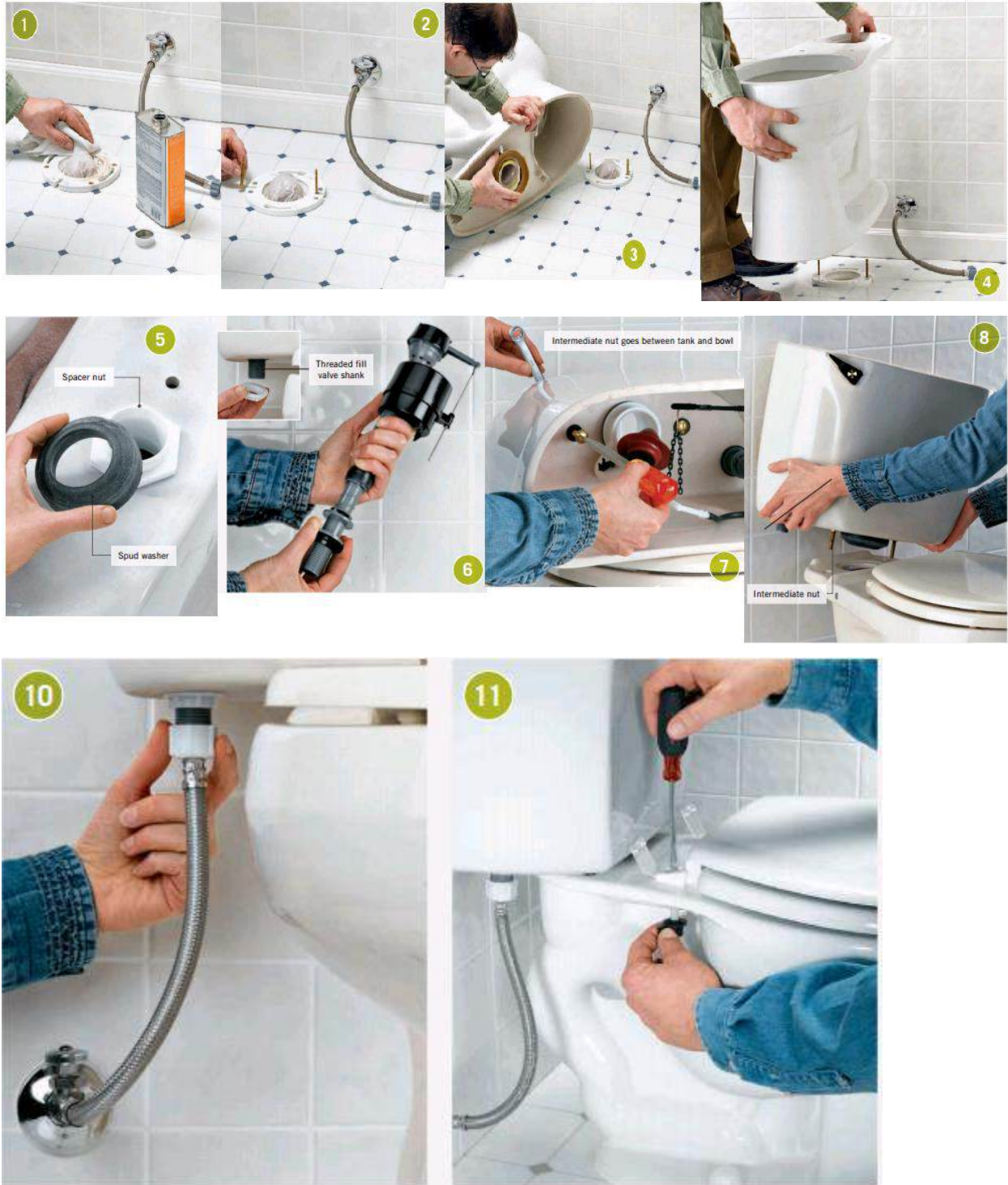
Figure 3.51 Steps installation of floor-mounted water closet bowl
