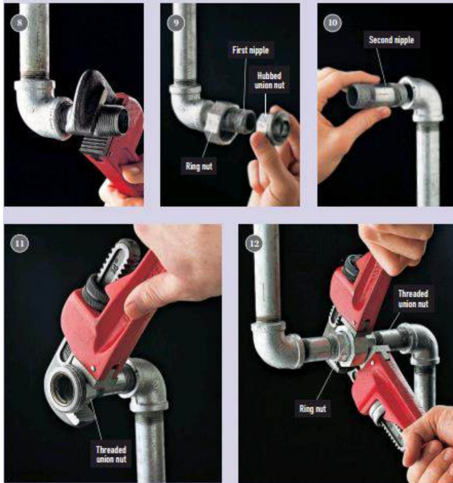
Figure 2.24 Replacing, maintaining, and joining old pipe
