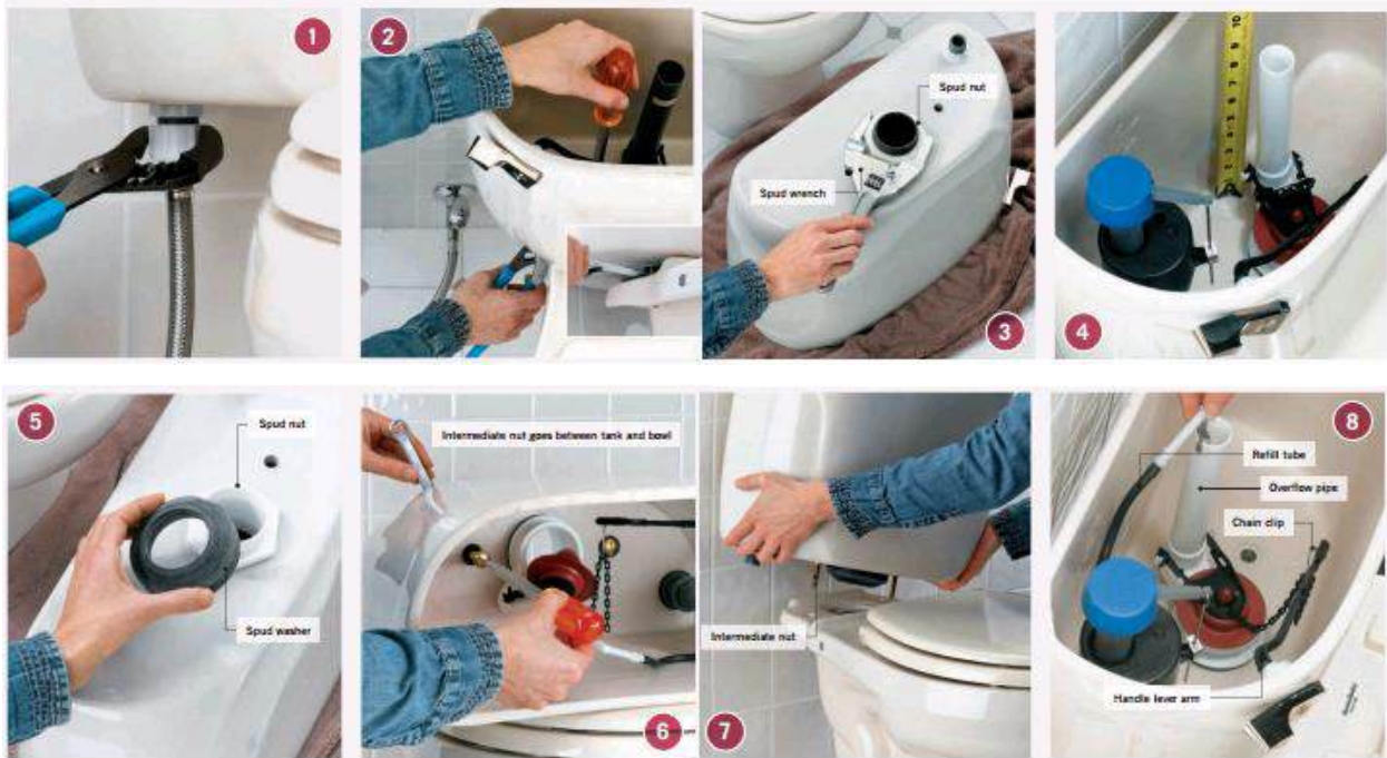
Figure 3.44 Installation of Flush Valve
