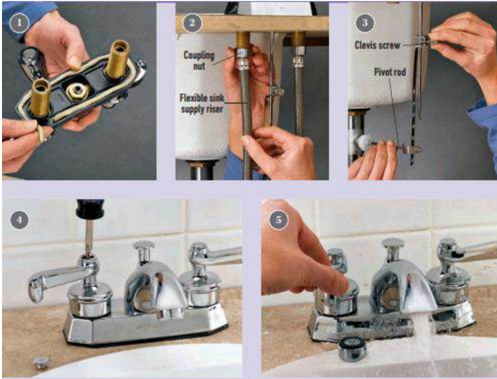
Figure 3.32 Installing a single-body faucet
