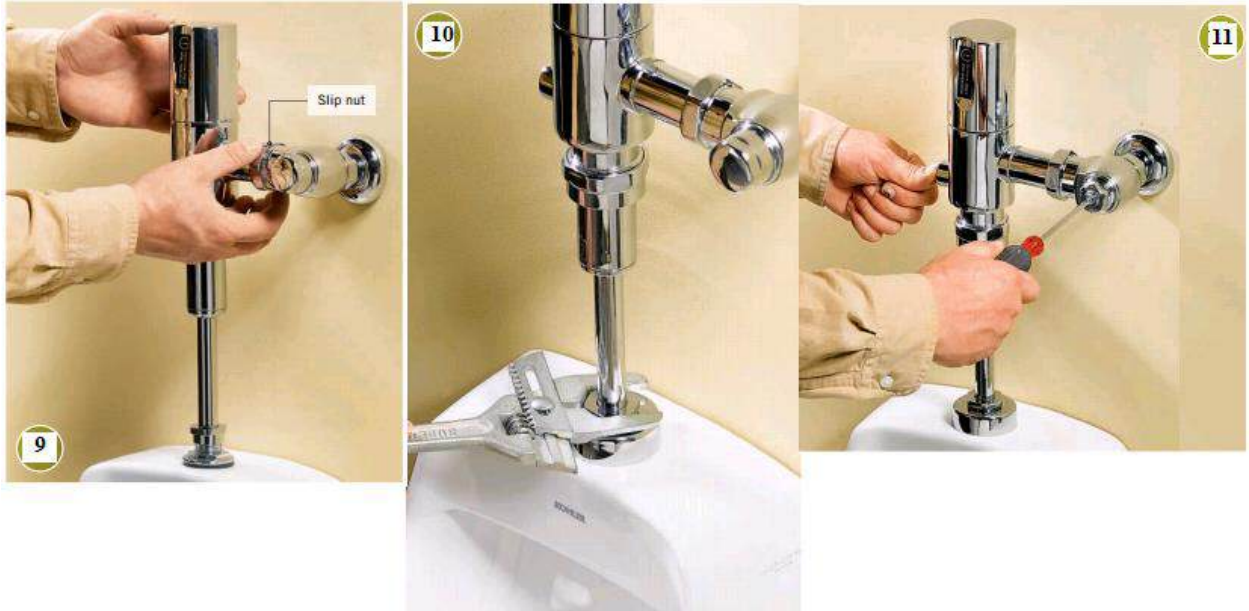
Figure 3.61 Steps to Install Wall-hung Urinal
