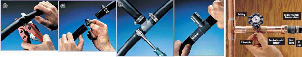
Figure 2.49 Steps to join flexible plastic pipe
