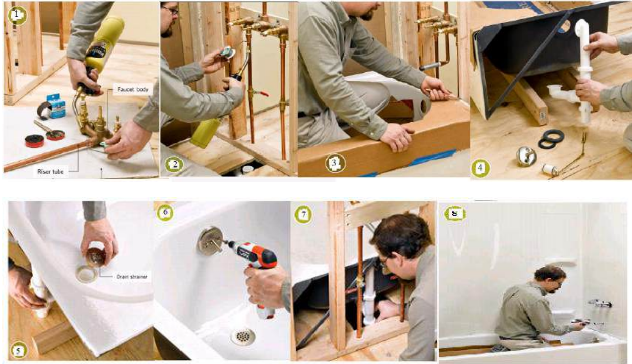
Figure 3.7 Steps of Installation of Bathtub
