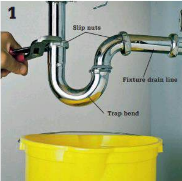
Figure 3.93 Remove and Clean Sink Drain Trap
