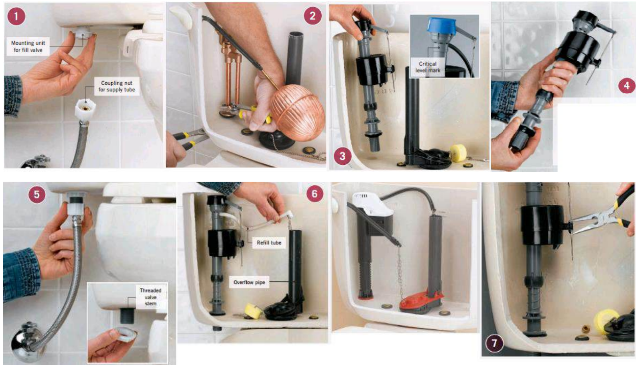
Figure 3.45 Installation of Fill Valve
