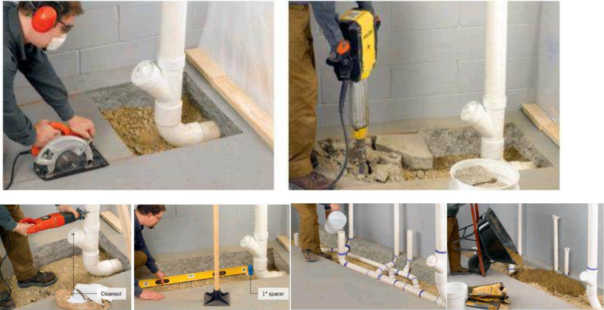
Figure 2.48 Steps of Installation of Basement Bath using rigid plastic pipe
