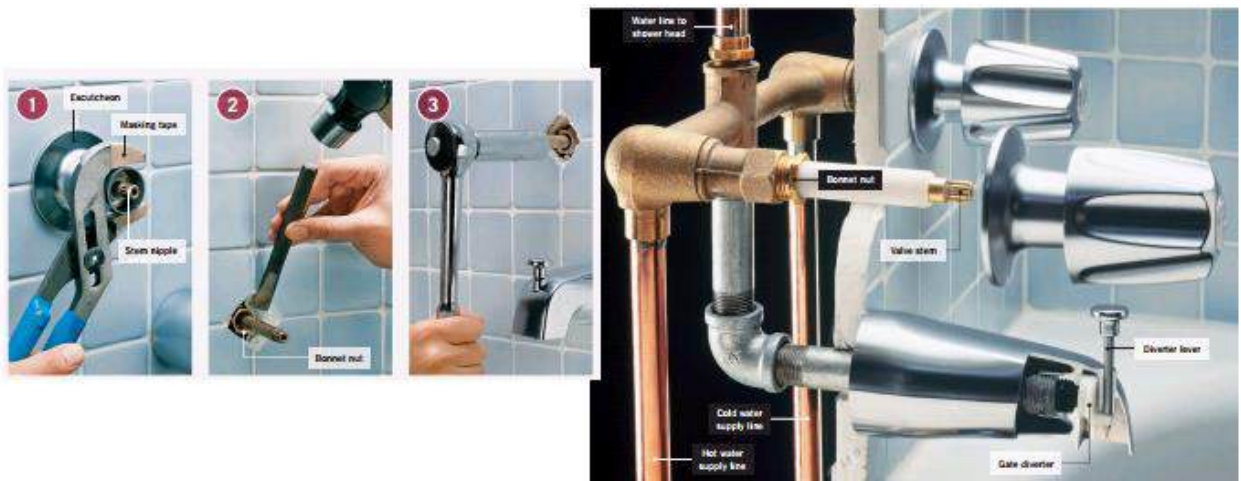
Figure 3.70 Fixing Three-Handle Tub and Shower Faucets
