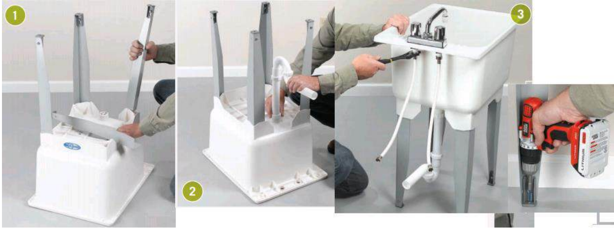
Figure 3.86 Detailed steps to install slop sink
