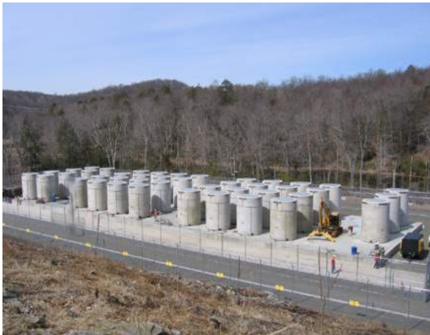
Figure 2-8: Dry storage at the Connecticut Yankee site (Source: Connecticut Yankee [17])
