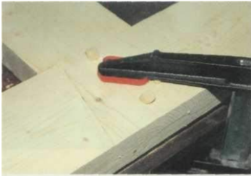
11 The dowels in place and the joint clamped.
