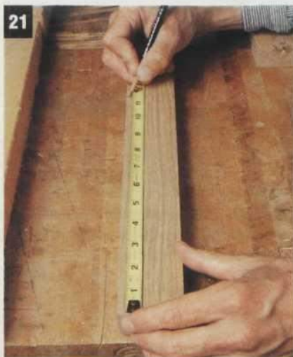
21 Measure an 11½" length on the 1" x 2" x 48" skirt piece. Square the mark and cut. Repeat for the remaining three skirt pieces. Now's the time to check the skirts and legs for blade burn, and sand the faces if needed.
