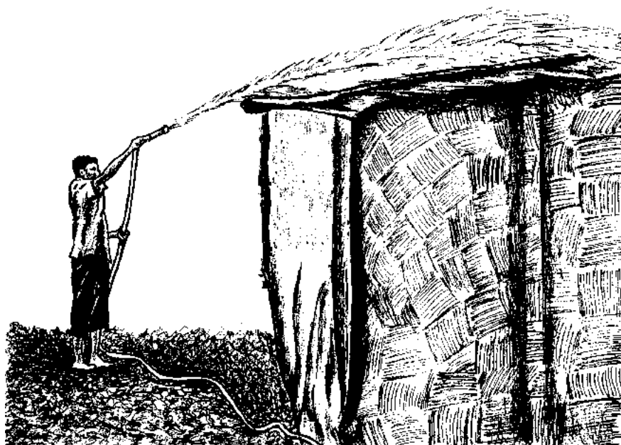
Figure 26: Spraying the jute-covered roof
