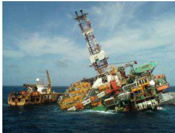
Figure 2.4.: The Petrobras P-36 oil platform sinking.
