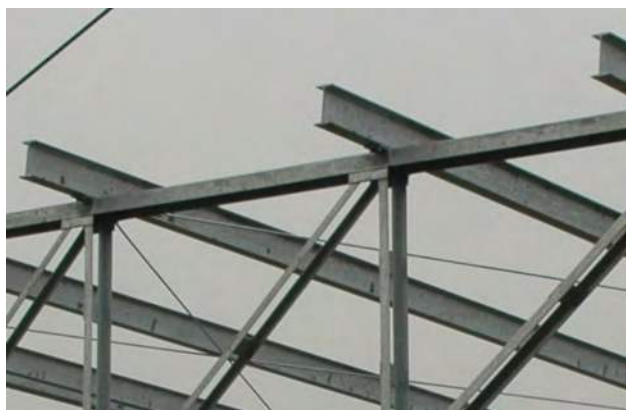
Figure 12.21 Steel I-beams are used in construction to reduce bending strains. (credit: modification of work by “US Army Corps of Engineers Europe District”/Flickr)
