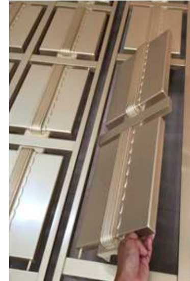
Fig 6.16 Detail of the liquid-metal coated aluminium facade screens
