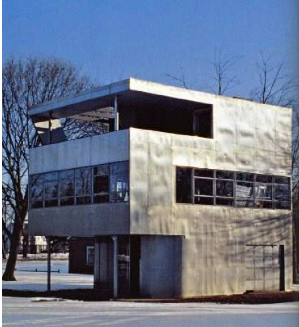
Fig 6.2 The aluminium clad Aluminaire House, architect A. Lawrence Kocher and Albert Frey, 1931
