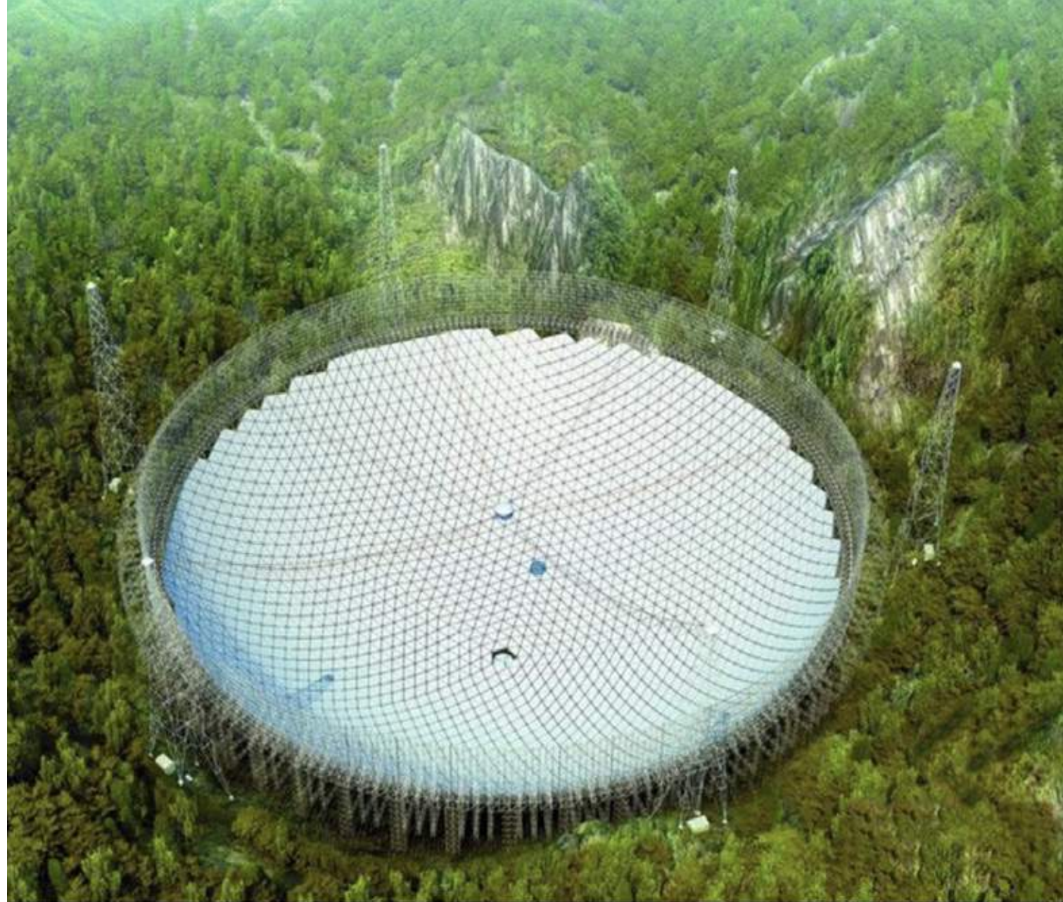
Fig 8.1 The Five Hundred Meter Aperture Spherical Radio Telescope, Pingtang, Guizhou, China, is skinned in perforated aluminium sheeting
