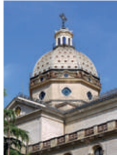
San Giocchino, architect Raffaele Ingami, 1897, the 1.3mm mill finished aluminium cladding of the dome of this church in Rome is performing well after nearly 120 years.
