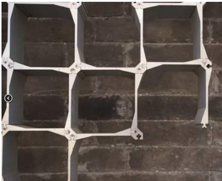
Fig 6.61 The interlocking anodised aluminium extrusions of the screens of Qianmen East, Beijing, China, architect Kengo Kuma & Associates, 2016
