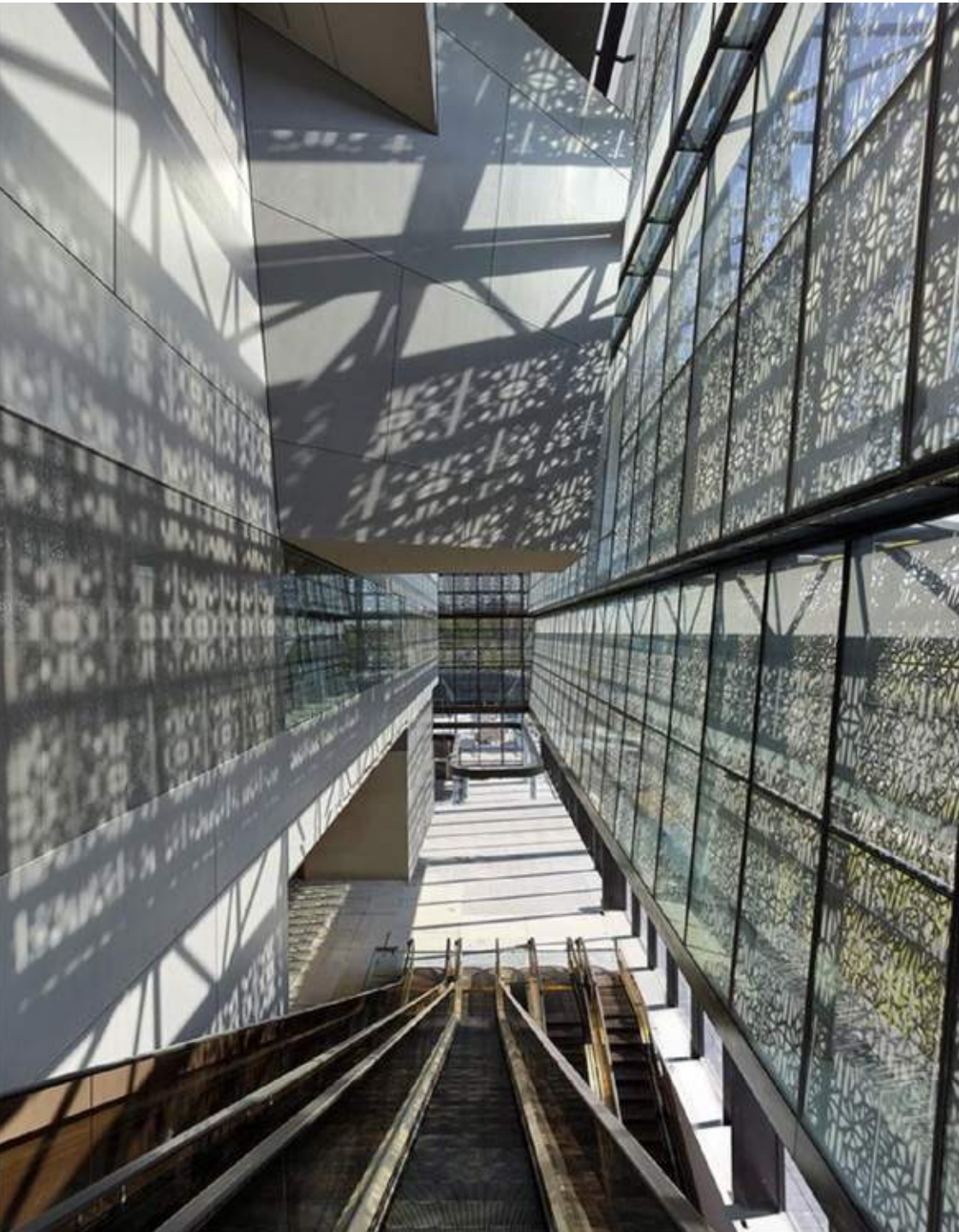
Fig 4.15 The dynamic shadows from the tracery of the cast aluminium cladding of the NMAAHC
