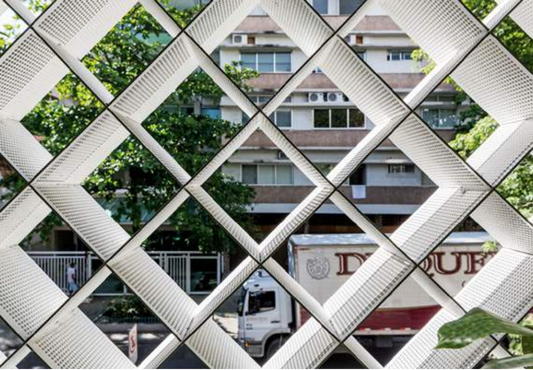
Fig 6.56 The view out through the aluminium perforated louvers of the Anibal Building, architect Bernardes Arquitetura, 2015
