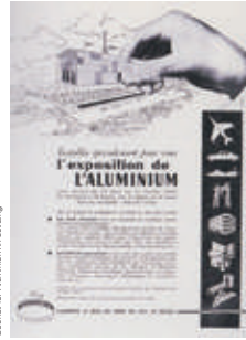
Aluminium Centenary Pavilion was designed by Jean Prouvé in 1954, this pavilion has now been assembled in three locations; banks of the Seine in Paris, Lille and now Paris Villeprinte.
