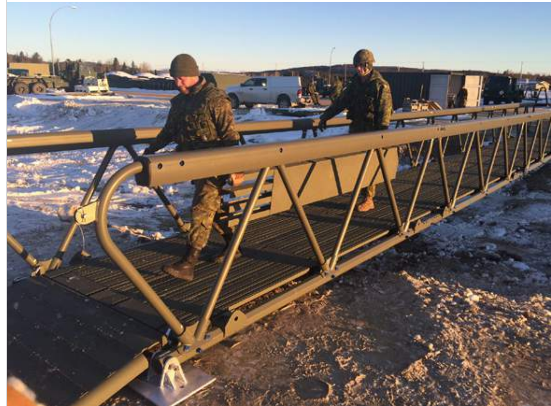
Fig 5.20 A prototype deployable military bridge, designed and fabricated in aluminium alloys by MAADI Group for the Canadian Army, 2017
