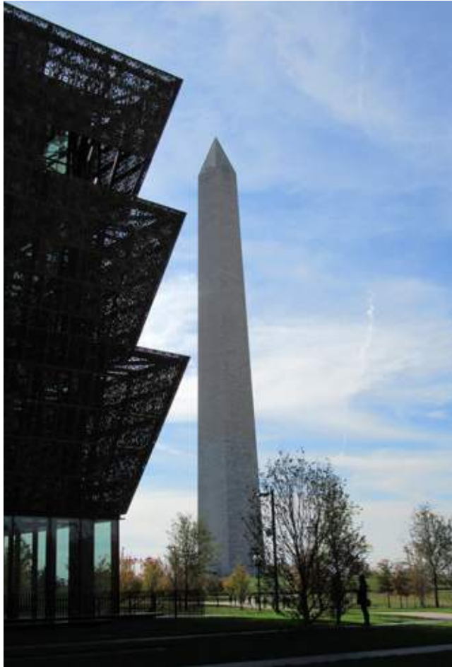
Fig 4.12 The inclined angle of the cast aluminium panels of the NMAAHC is a direct inversion of the 17° pyramidal cast aluminium cap of the Washington Monument.
