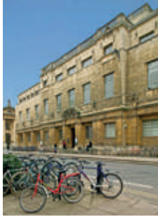
The anodised aluminium windows of New Bodleian Library, Oxford, architect Sir Giles Gilbert Scott, 1938 – are due to last another 60 years.
