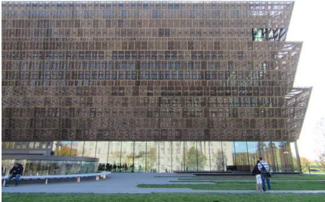
Fig 4.10 The cast aluminium panels on the north façade of The National Museum of African American History & Culture
