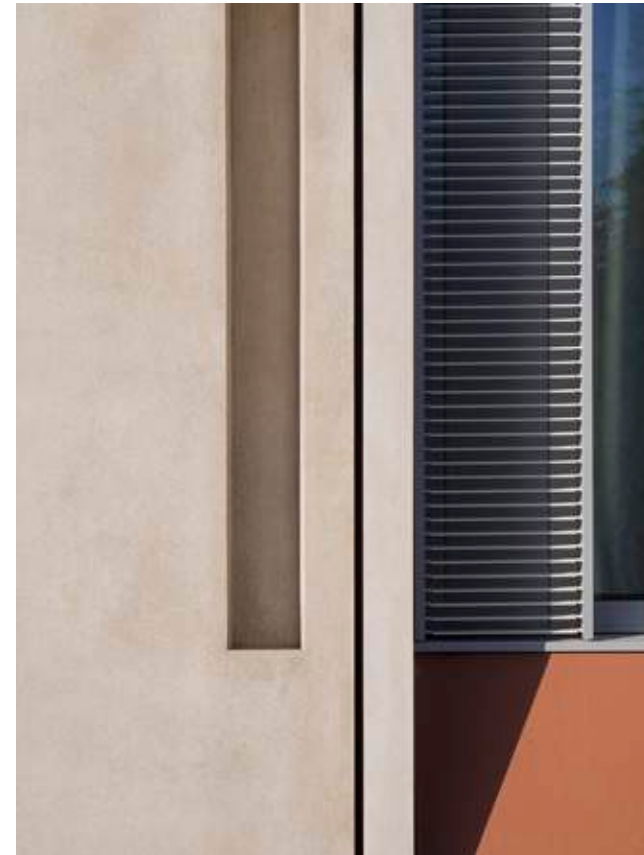
Fig 5.8 Ash Court, thermally broken triple glazed aluminium window, louvers and precast concrete
