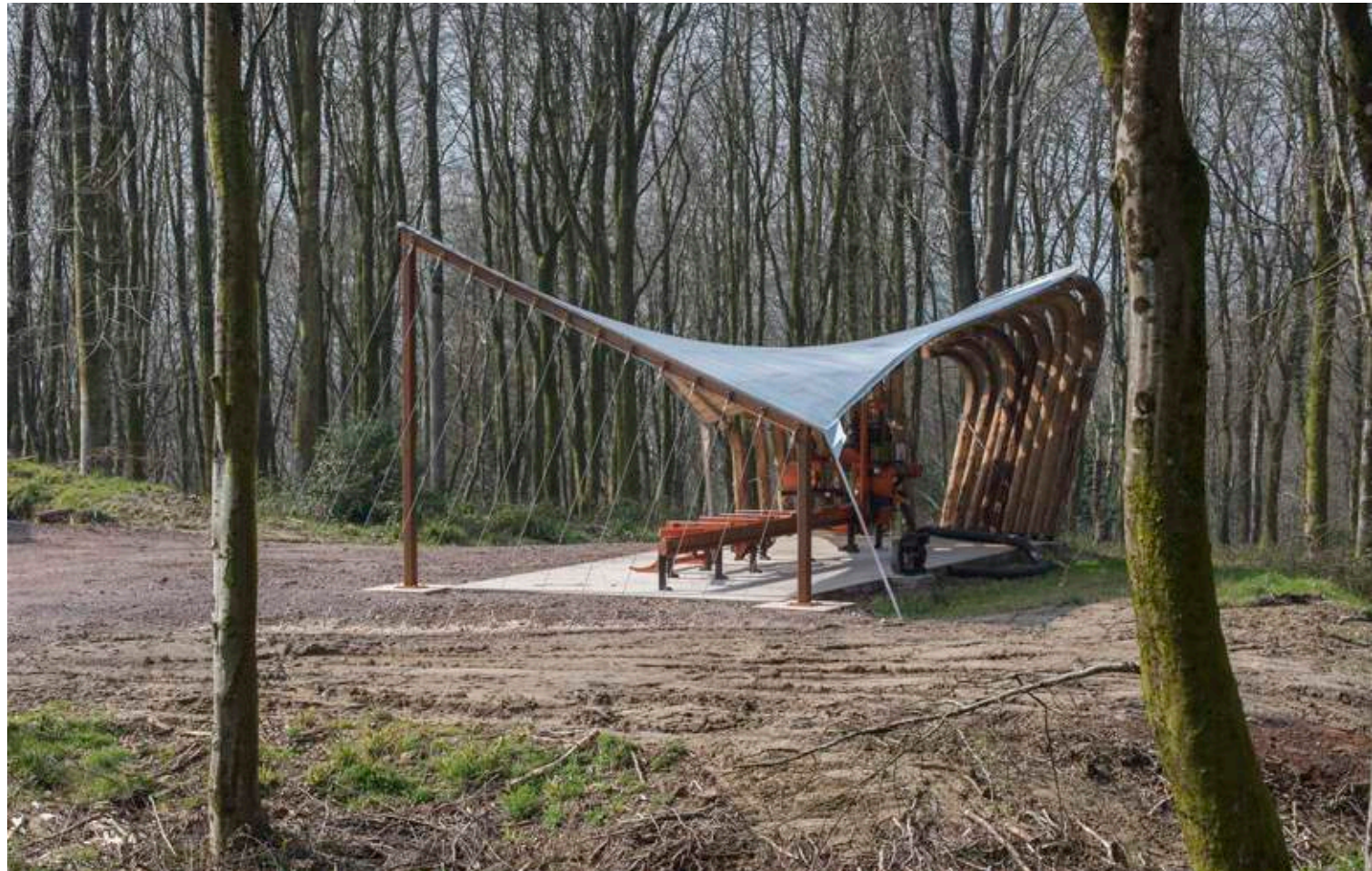
Fig 6.69 Sawmill Shelter, Hooke Park, England, designed and built by AA Design + Make Students, 2016
