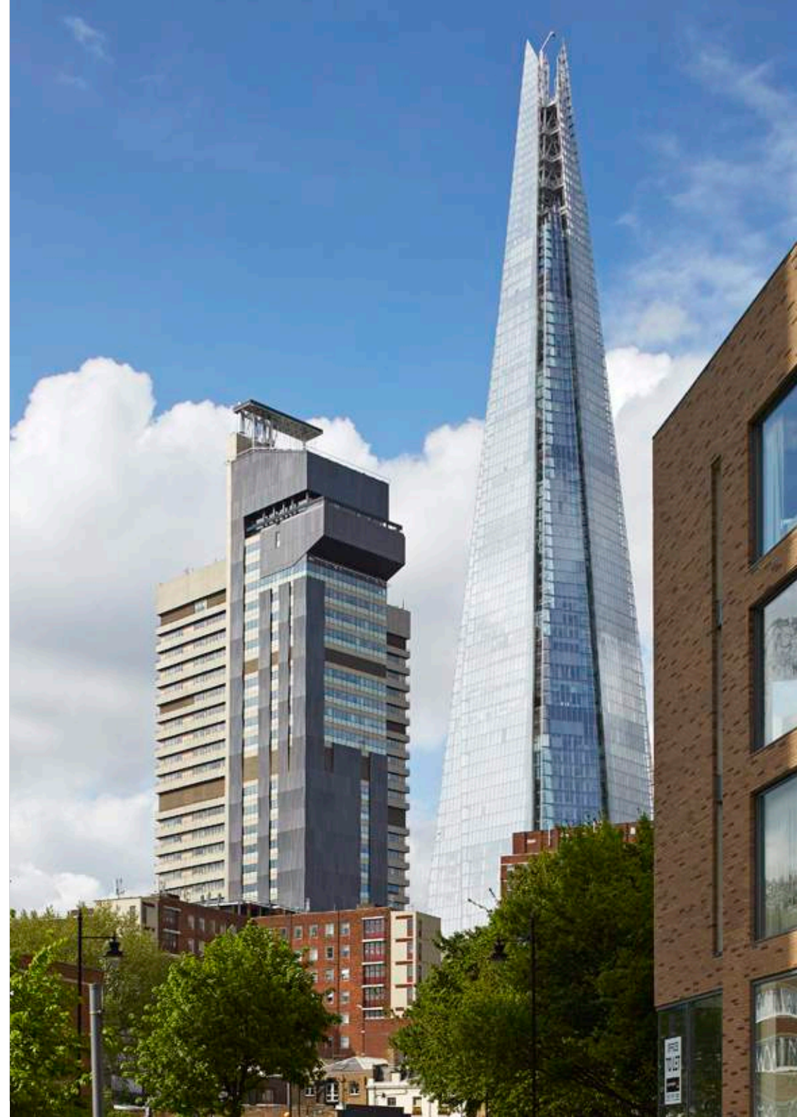
Fig 1.16 Guy's Hospital overcladding designed by Penoyre & Prasad and the Shard, designed by Renzo Piano Building Workshop: have equally durable but distinct finishes on their aluminium building envelopes – anodising and Class 2 polyester powder coating
