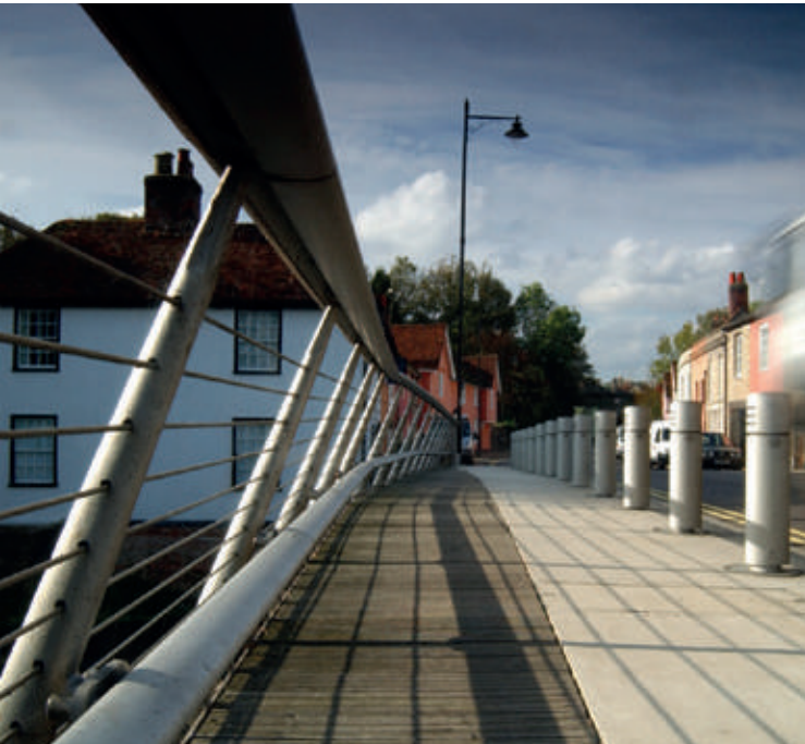
Aluminium has many qualities that make it ideal for use within architecture and the built environment - it is: Durable, Recyclable, Flexible, Light and Strong, Powerful, Economic and Sympathetic. Ballingsdon Bridge, Suffolk, designed by Michael Stacey Architects, 2003. The pedestrian handrails, assembled with bespoke aluminium extrusions, are capable of stopping a 42 tonne truck.
