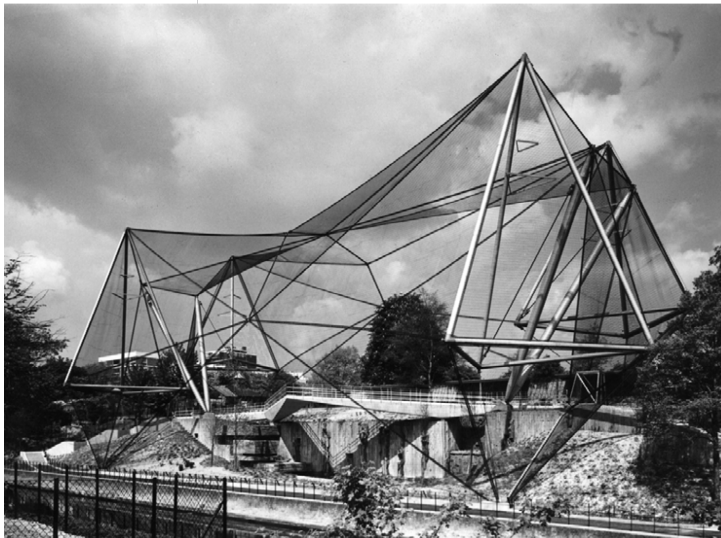
Fig 8.35 The Snowdon Aviary, with its tubular aluminium alloy structure, at Regent's Park Zoo, architect Cedric Price with engineer Frank Newbery and detailed input from Lord Snowdon, completed in 1965. The Snowdon Aviary is Grade II* listed by Historic England (13223695). In 2017 Foster + Partners are in the process of restoring this enclosure and converting to house Colobus monkeys
