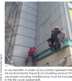
Guy's Hospital Tower, London, architect Penoyre & Prasad, 2014. This anodised aluminium over cladding and reglazing of the world's tallest hospital tower has a carbon pay back period of less than 13 years.
