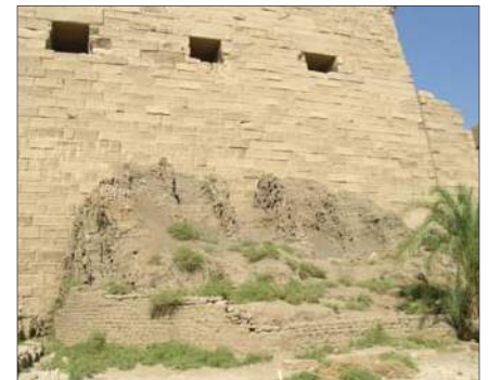
The mud brick ramp used in the construction of pylon I can still be seen today.
