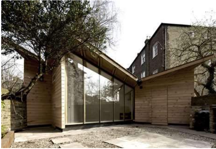
Fig. 52 The saw-toothed frontelevation which maximises natural daylight and passive solar heating to the interior.
