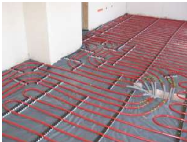
Fig. 60 Underfloor heating pipes, before they are covered by the screed
