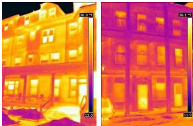
Fig. 97 Thermal photo of a building
