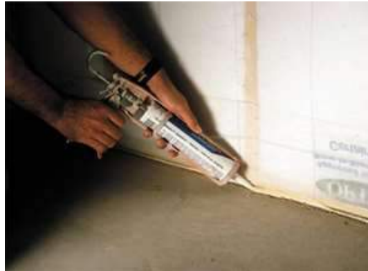
Fig. 55 Caulking the cracks
