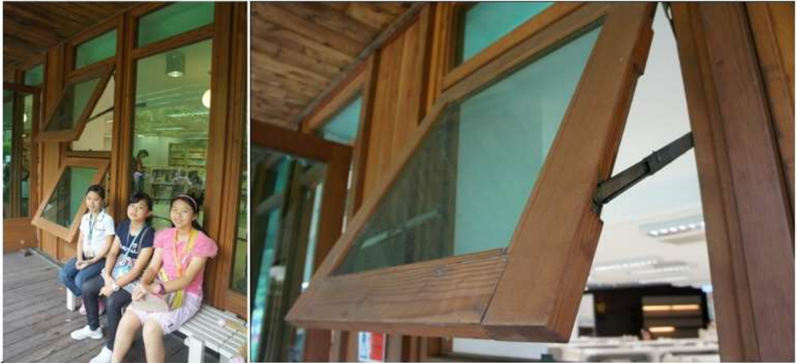
Fig. 136 Example of air flow control
