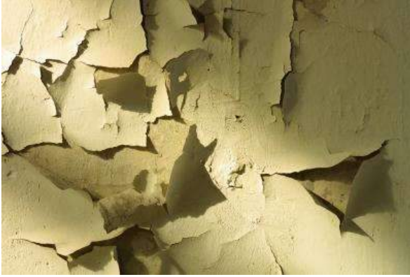
Fig. 74 Peeling paint
