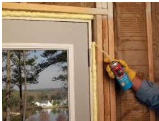
Fig. 56 Closing a gap between window frames and outside wall
