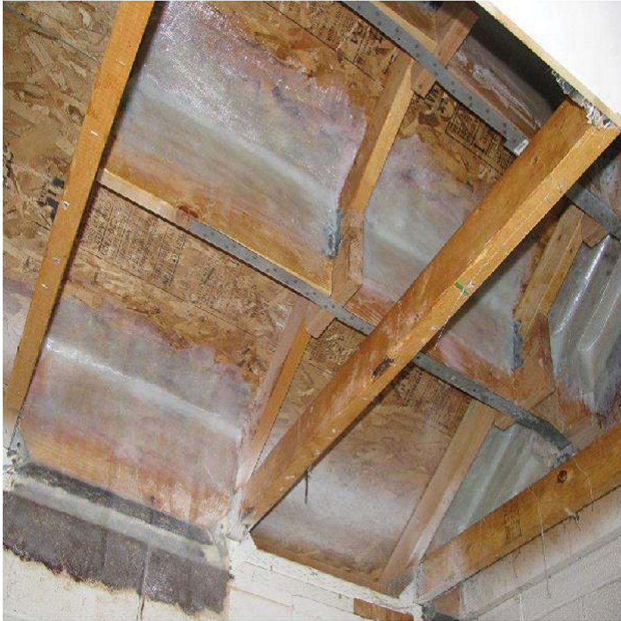
Fig. 4 Typical installation of FRP in a wood roof system
