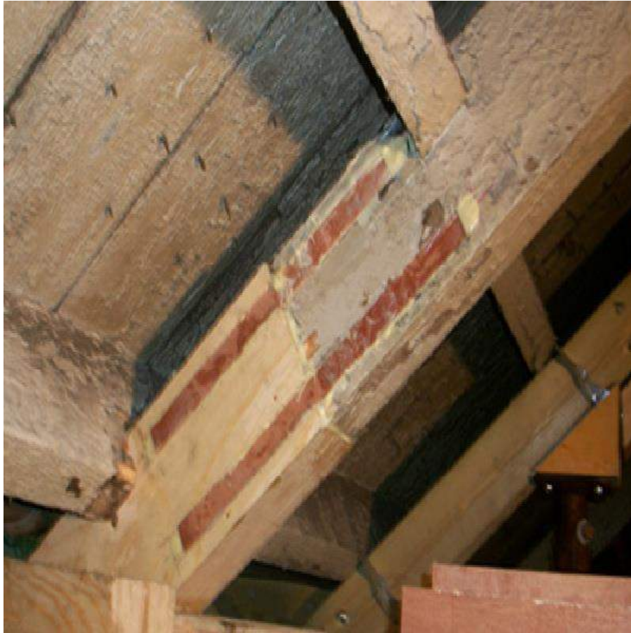
Fig. 5. Repair wood structures with epoxy resins
