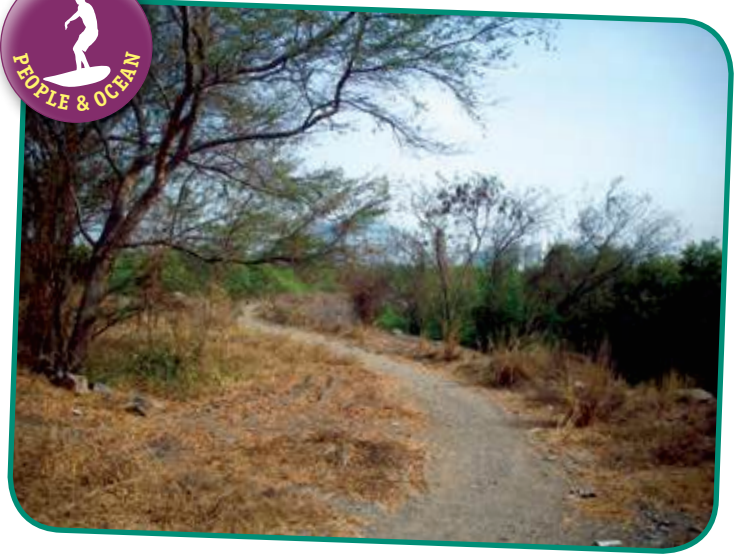
A ROAD CONSTRUCTED THROUGH THE VASHI MANGROVE FORESTS. THESE MANGROVE FORESTS ARE ALSO BEING USED TO DUMP WASTE, GRADUALLY DEGRADING THE RICH FORESTED LAND AND ITS UNIQUE WILDLIFE INTO WASTELAND ONLY FIT FOR CONSTRUCTION. © Rudolph A. Furtado, WMC
