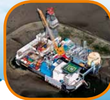
GERMANY'S LARGEST OIL FIELD MITTELPLATE. © Ralf Roletschek, WMC
