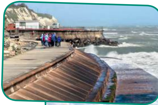
A SEAWALL IN VENTNOR, ISLE OF WIGHT. © Oikos-team, Wikipedia
