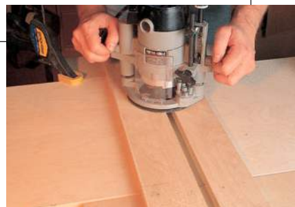
Here's the simple jig to rout the dados. It uses a bearing-on-top straight bit to guide against the edges of the jig. Clamp the jig right on the marked lines and rout the dado.
