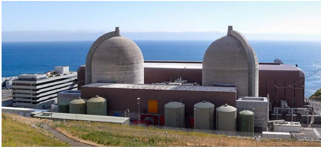
Figure 6 Example of a larger reactor: the two-unit Diablo Canyon nuclear power plant
