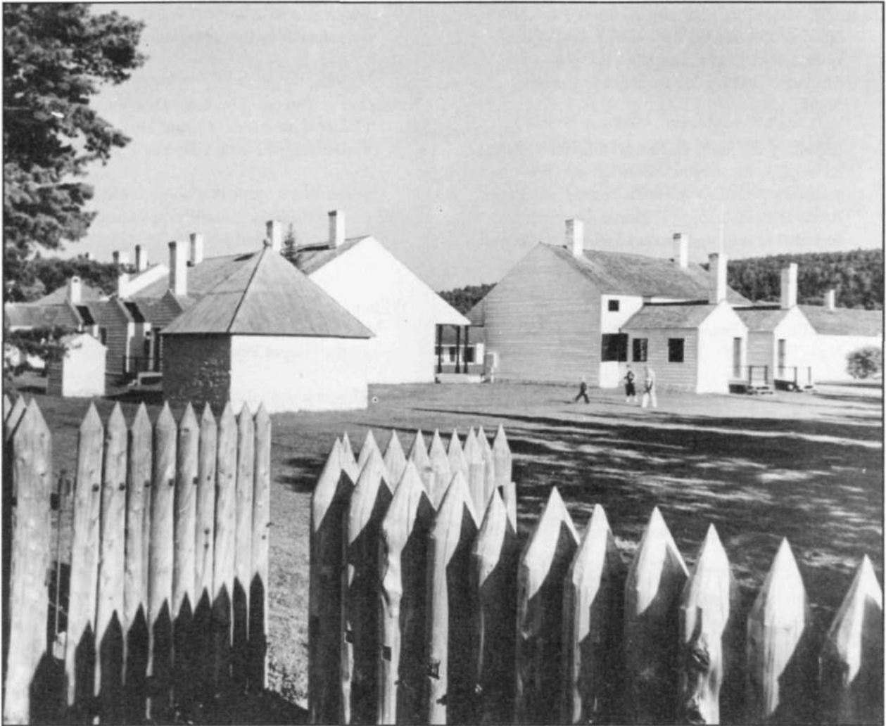
Wood was used not only for the pointed log stockade, but also for the majority of the structures erected in the 1840s at Fort Wilkins in Copper Harbor, Michigan. Most of the garrison buildings are constructed of hewn logs, covered with clapboards. Photo: National Park Service files.
