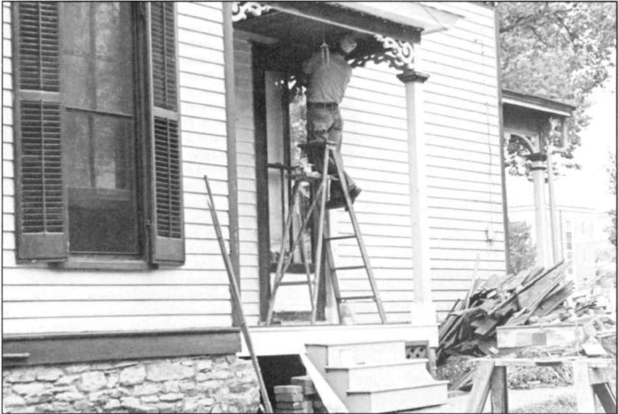
Restoration or replacement of deteriorated wood features usually requires the skill of a professional carpenter. Photo: Nebraska State Historical Society.
