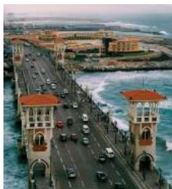
Ponte Stanley - Alexandria
